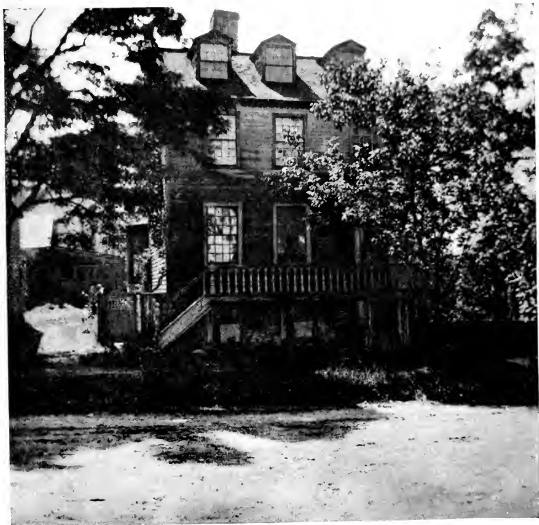
THE OLD GOVERNOR'S HOUSE, SHELBURNE.
