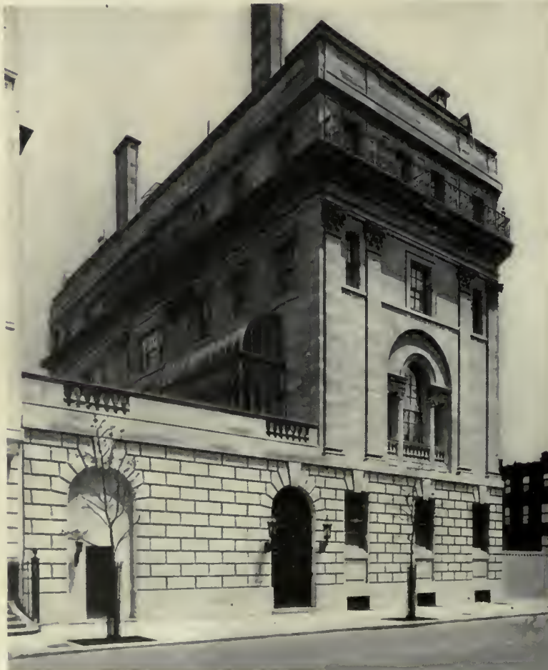
General View from the Street
