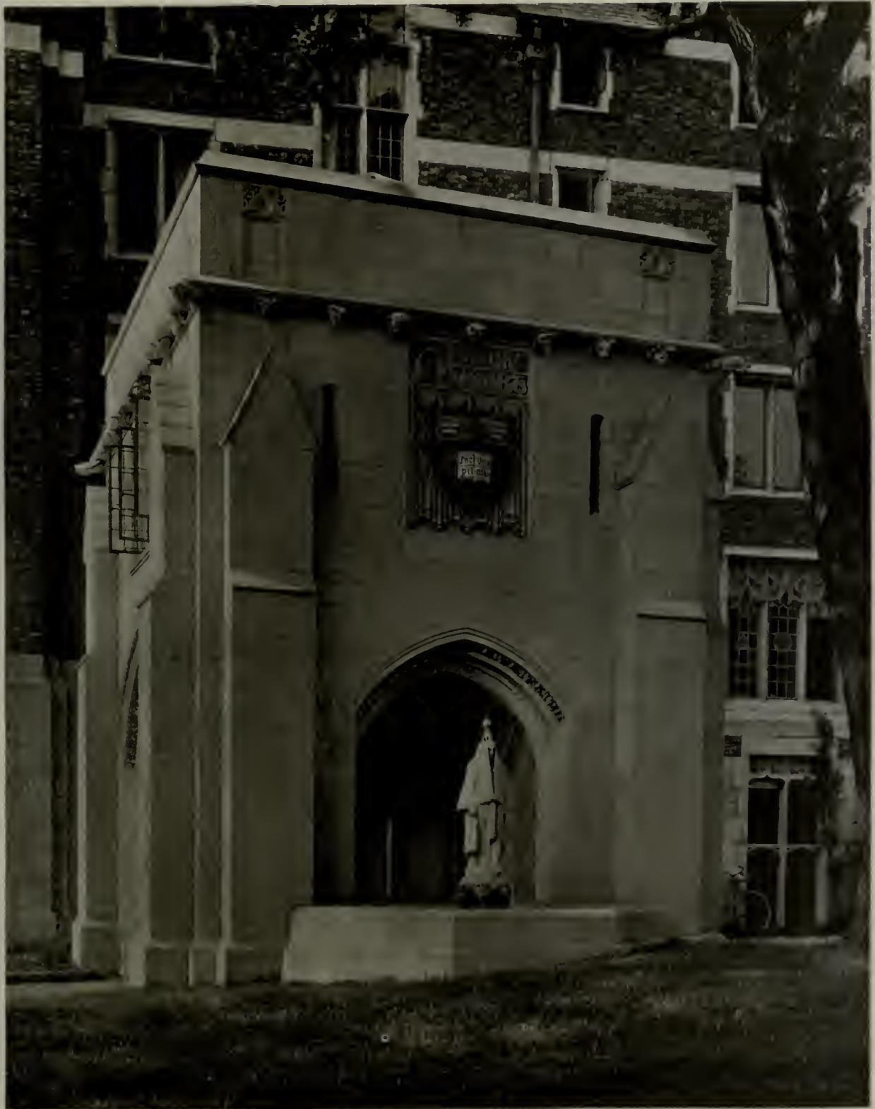
PORTE COCHÈRE AND FOUNTAIN, TOWER COURT DORMITORIES FOR WELLESLEY COLLEGE, WELLESLEY, MASS. COOLIDGE & CARLSON, ARCHITECTS
