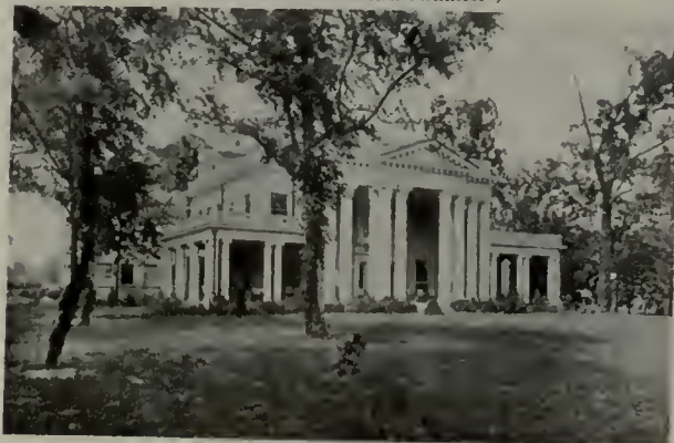
House for M. C. Heath, Esq., Columbia, S. C. Edwards & Sayward, Architects
