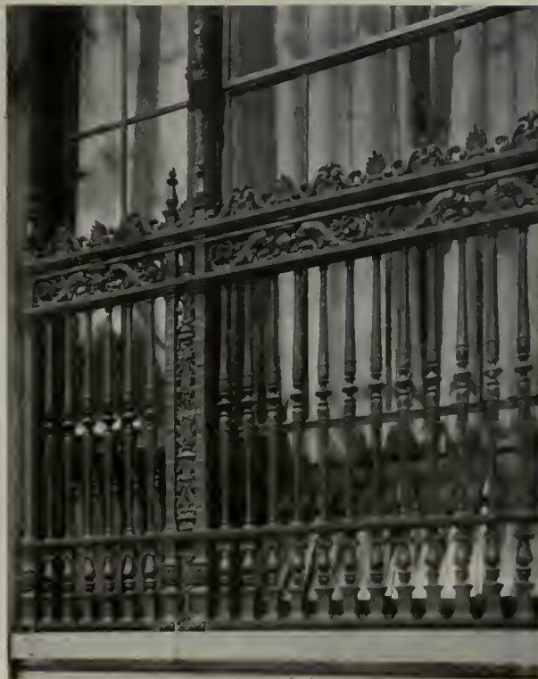
Detail of Window Grille
