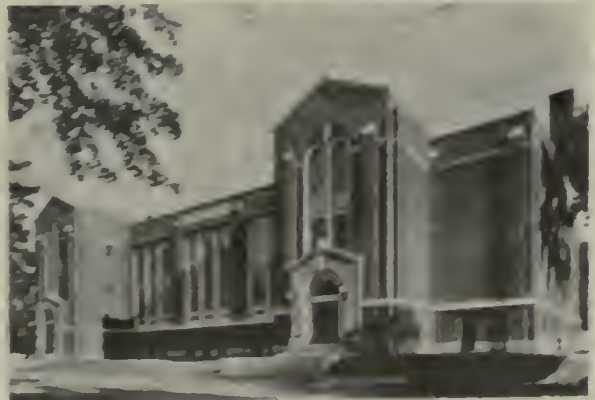
Baldwin High School, Birmingham, Mich. VanLeyen & Schilling, Architects. H. J. Knough, Associate
