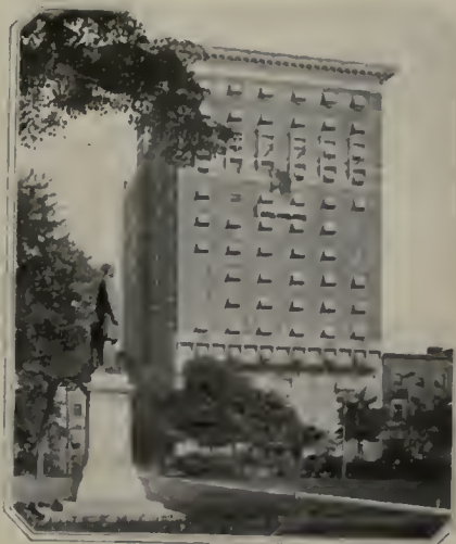
Robert Treat Hotel, Newark, N. J.; Gulsberg & Betelle, Architects; Crane Company, Newark, N. J., Jobbers; Jahnig & Peoples, Plumbers
