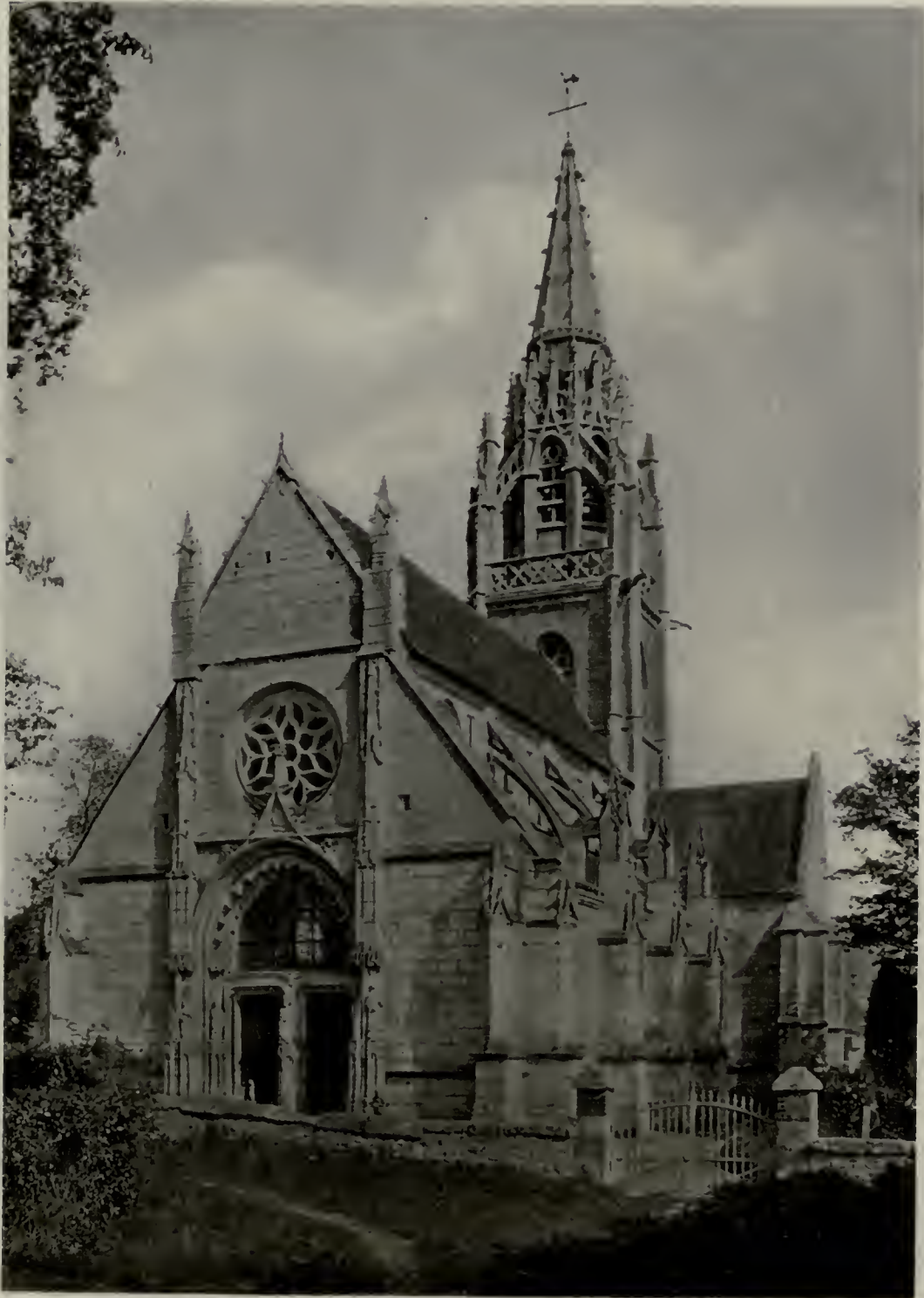
CHURCH AT VILLERVILLE
