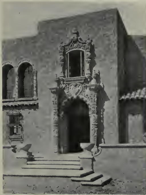
Entrance, Residence of George C. Rew, Esq. Coronado, Cal. Elmer Grey, Architect
