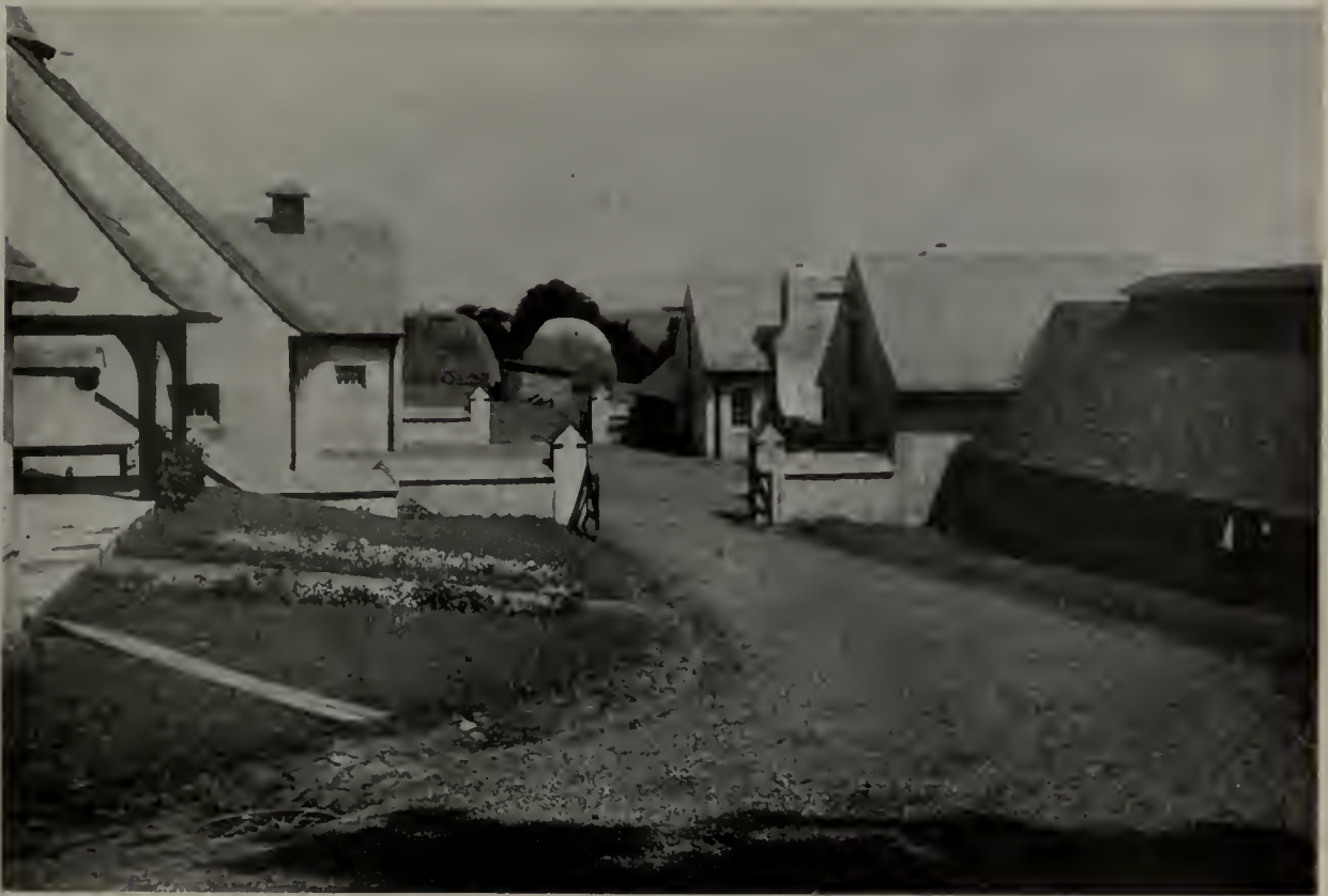
Lower Level from the West
