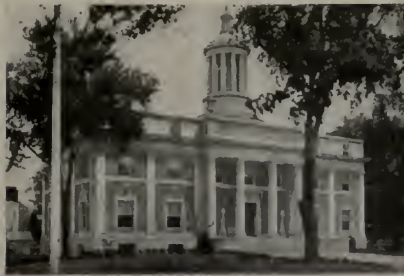
Municipal Building, Plainfield, N. J. Laurence F. Peck, Wm. Lawrence Bottomley Associate Architects
