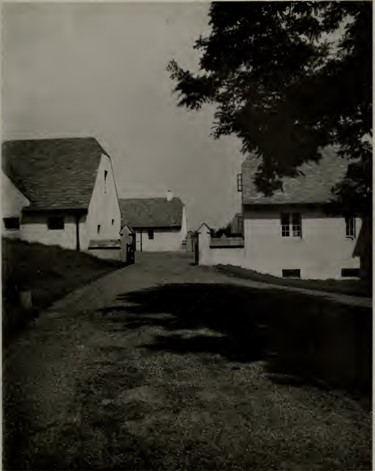
THE UPPER LEVEL FROM THE WEST
