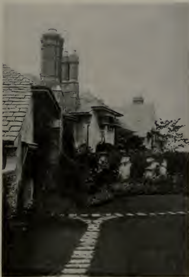
Entrance Front from the South-west
