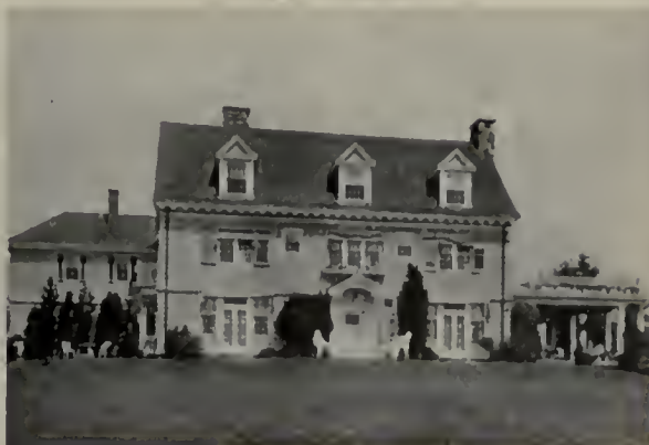
Country House, Far Hills, N. J. Emilio Levy, Architect
