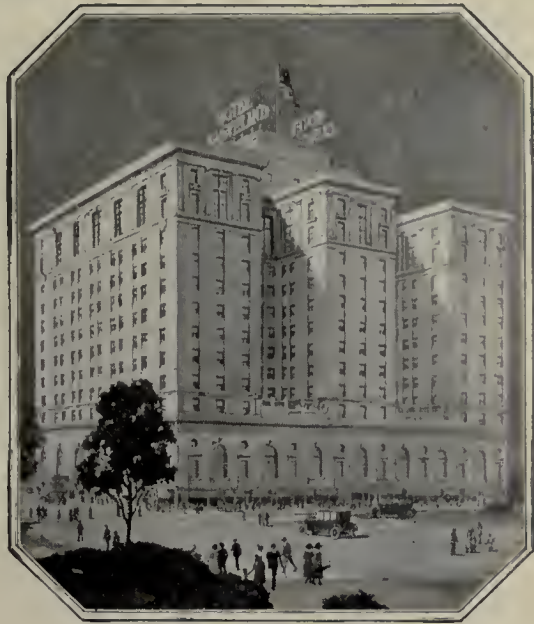
Hotel CLEVELAND Ohio: Graham, Anderson, Probst & White, Chicago, Architects; John Simmons Co., New York, Jobbers; W. G. Cornell Co., New York, Plumbers.
