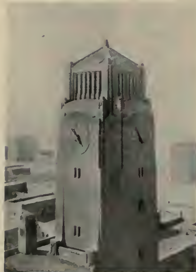
Tower, Pennsylvania R. R. Freight Terminal, Chicago, Ill. Price & McLanahan, Architects
