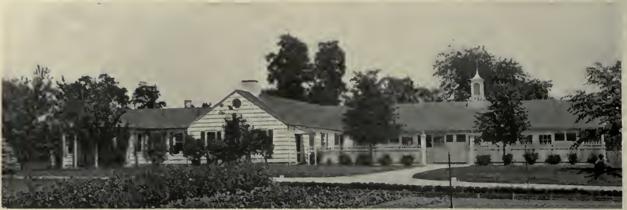
Farm Buildings on the Estate of Glenn Stewart, Esq., Locust Valley, L. I.
