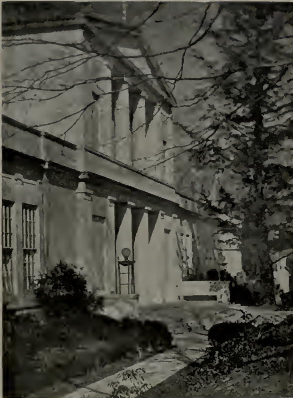
School for Frank A. Vanderlip, Esq., Scarborough, N. Y. Welles Bosworth, Architect
