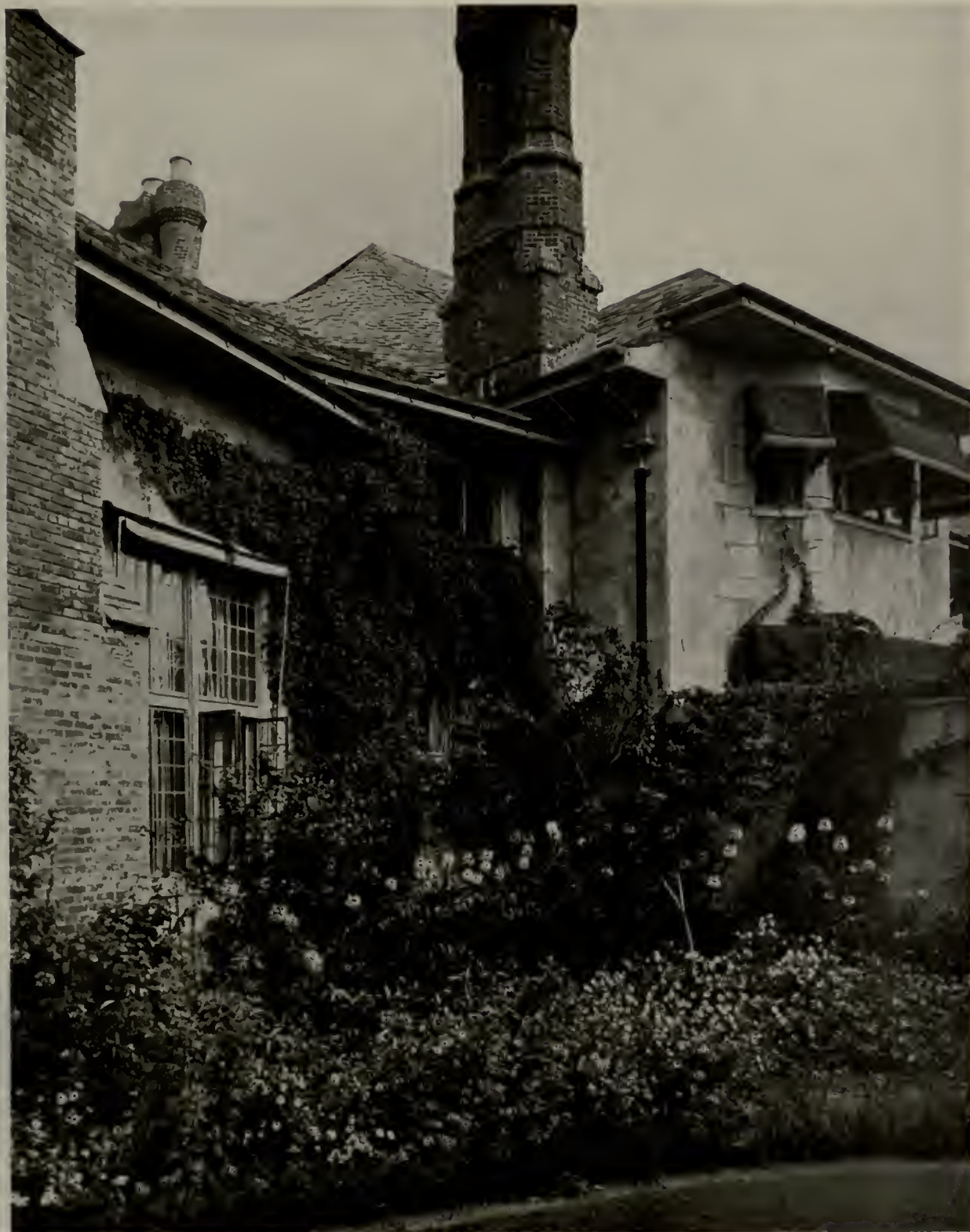
JUNCTION OF LIVING ROOM WING AND MAIN BUILDING RESIDENCE FOR CHARLES H. SABIN, ESQ., SOUTHAMPTON, L. I. CROSS & CROSS, ARCHITECTS
