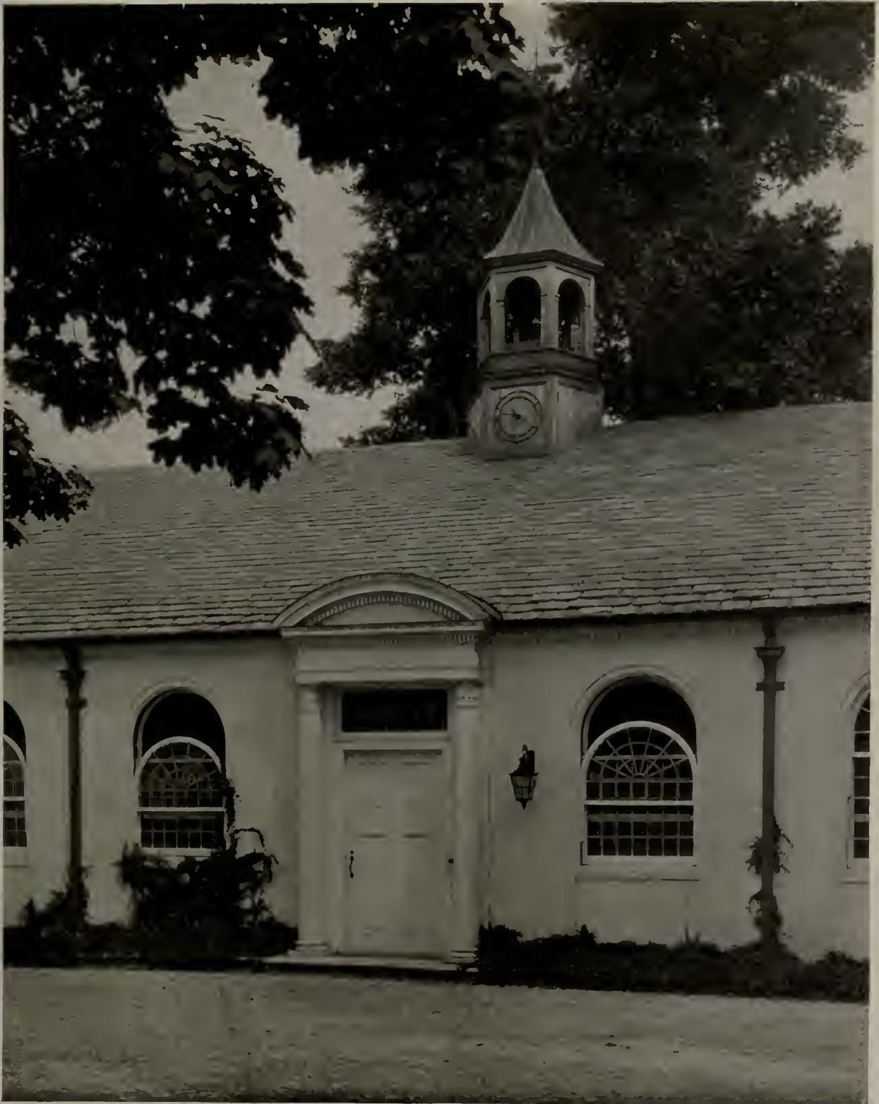
DETAIL OF RIDING ACADEMY HOUSE FOR W. R. GRACE, ESQ., WESTBURY, L. I. JAMES W. O'CONNOR, ARCHITECT
