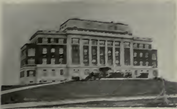
Carson C. Peck Memorial Hospital, Brooklyn, New York City Ladlow & Peckoby, Architects
