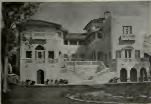
House for Charles L. Briggs, Miami, Fla. Condon E. Miner, Architect
