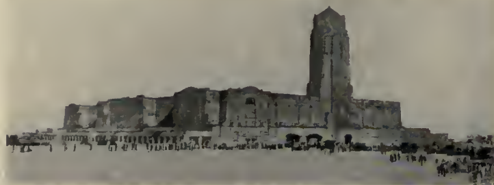
Pennsylvania R. R. Freight Terminal, Chicago, Ill. Price & McLanahan, Architects
