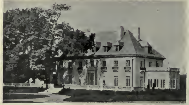
Residence of Henry I. Harriman, Esq., Newton, Mass. John Barnard, Architect
