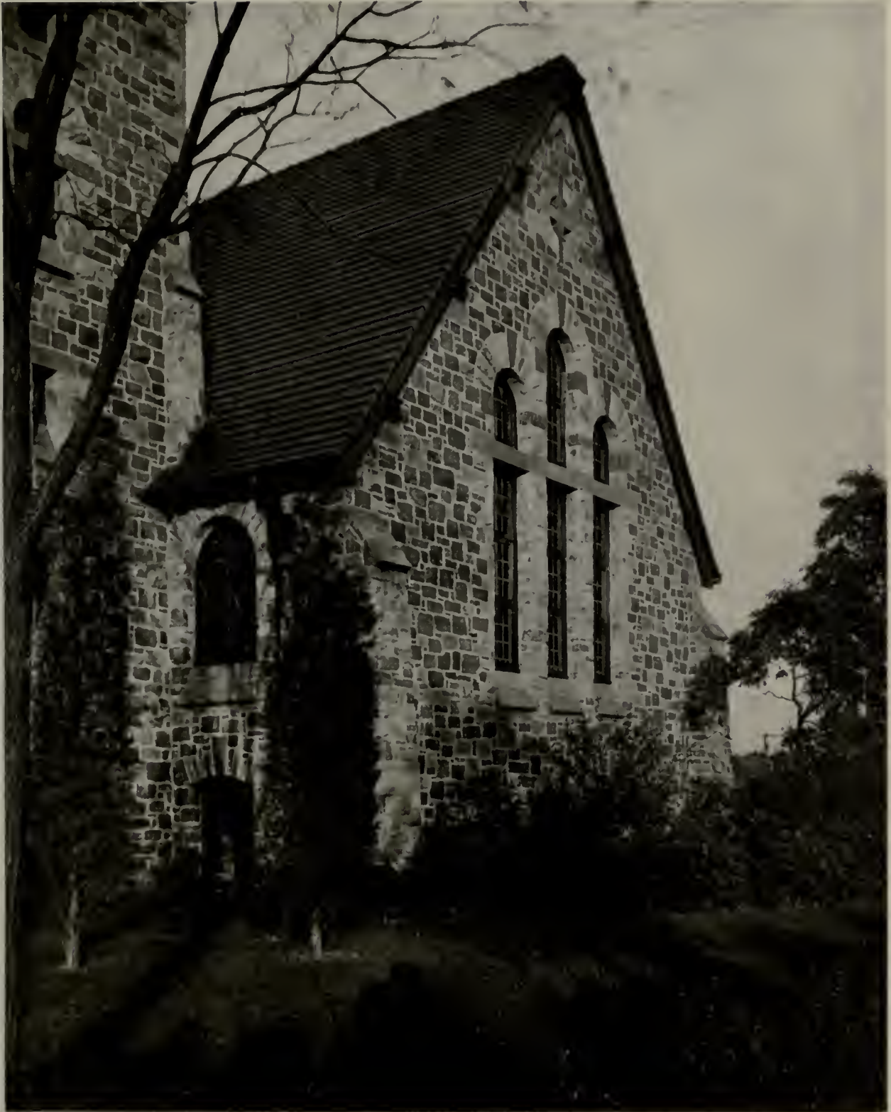
VIEW FROM THE SOUTHWEST
