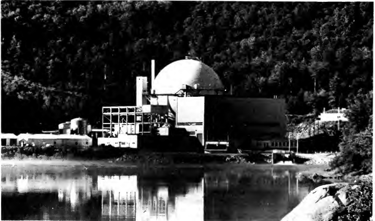
The Yankee Atomic Electric nuclear power station in Rowe, Massachusetts.
