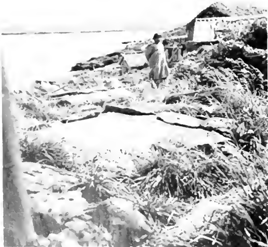
FIG. 63. Gut window of house resting on wooden framework and held in place by large, flat stones.
