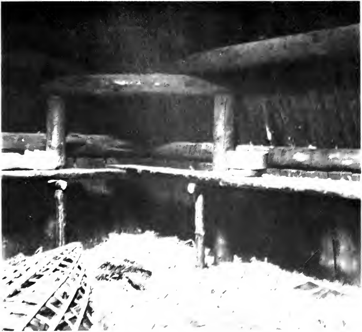
FIG. 65. Corner of a qasgiq showing cribbed roof on two of the eight supporting posts. Men sat on floor and children on high benches above them. There is a wooden urine tub on the bench.
