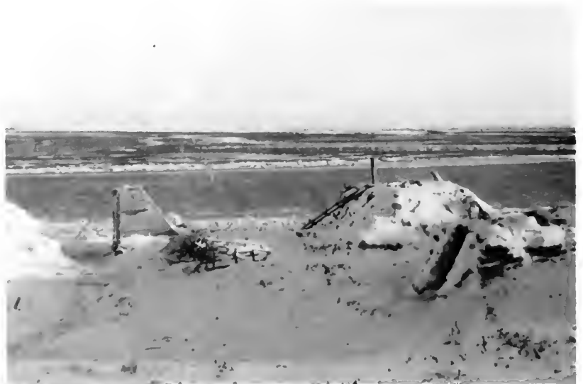
FIG. 64. House with roofed underground entrance passage through which one moved in a stooping posture and with the outer door modeled after a ship's companionway. House entrance at right is of older type.
