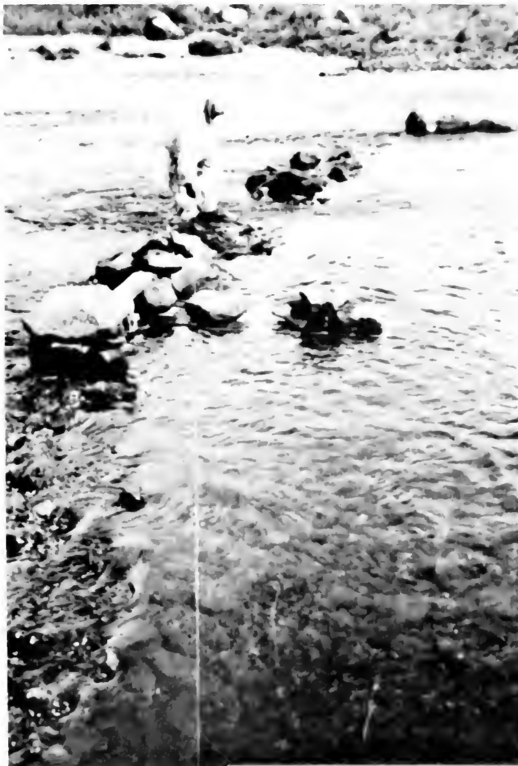
FIG. 29. Constructing a dam with an opening left for fish traps.
