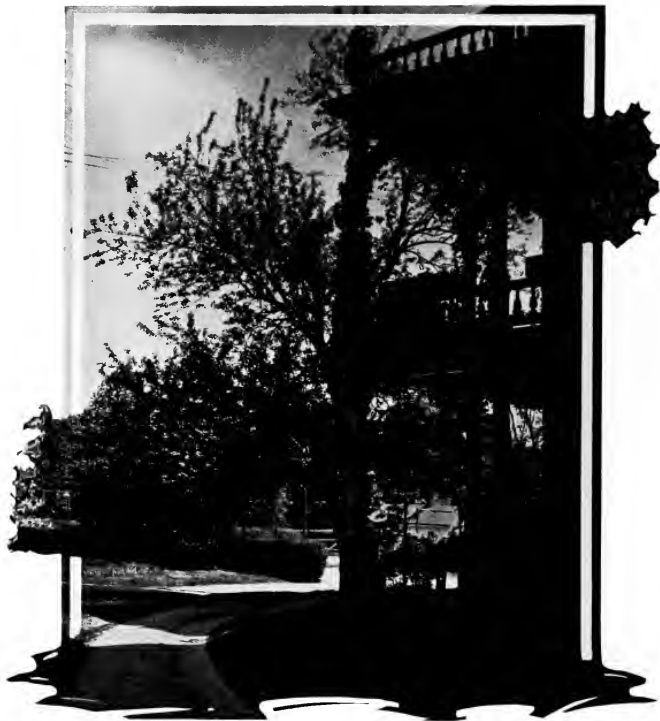
CORNER OF MAIN BUILDING
