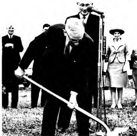
The library gets its start with Dr. Campbell at the shovel.
