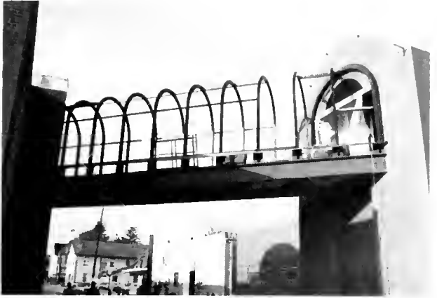
An overhead bridge joins the main building to a smaller structure, which formerly housed the Co-op Store.
