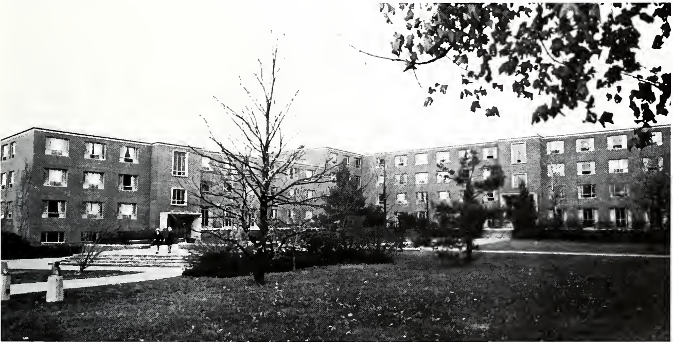
The oldest on-campus dormitory in use, Woody Hall housed its girls within its sprawling architecture of varied levels and sections.
