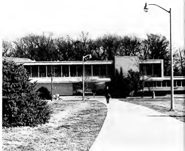
The Agriculture Building was constructed by the University to allow further agricultural research projects.
