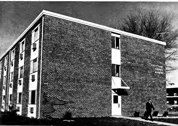
Egyptian Sands living area is composed of efficiency apartments and includes four buildings housing both men and women.
