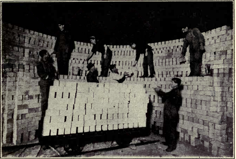
FIG. 1.—Interior view of circular down-draft kiln. (Photo loaned by Robinson Clay-product Manufacturing Co.)
