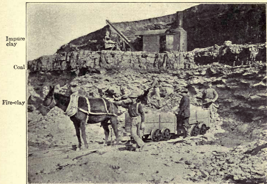
FIG. 1.—Section showing fire-clay underlying coal-seam. The upper clay above coal is of impure character. (Photo loaned by Robinson Clay-product Company.)
