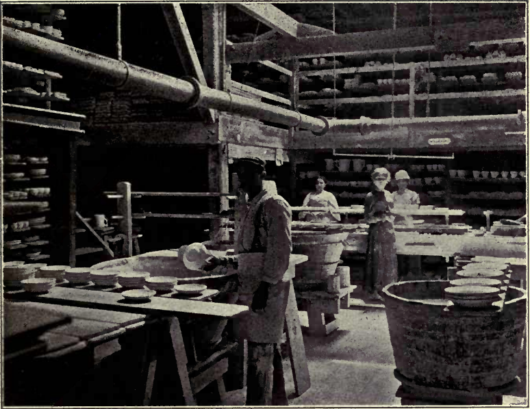
Dipping biscuit ware into the glazing-tubs. (Photo by H. Ries.)
