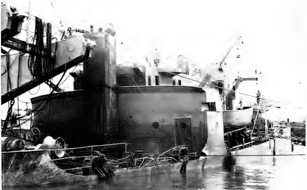
The USNS Kellar (T-AGS 25), a victim of Hurricane Betsy, is salvaged from the Mississippi River.
