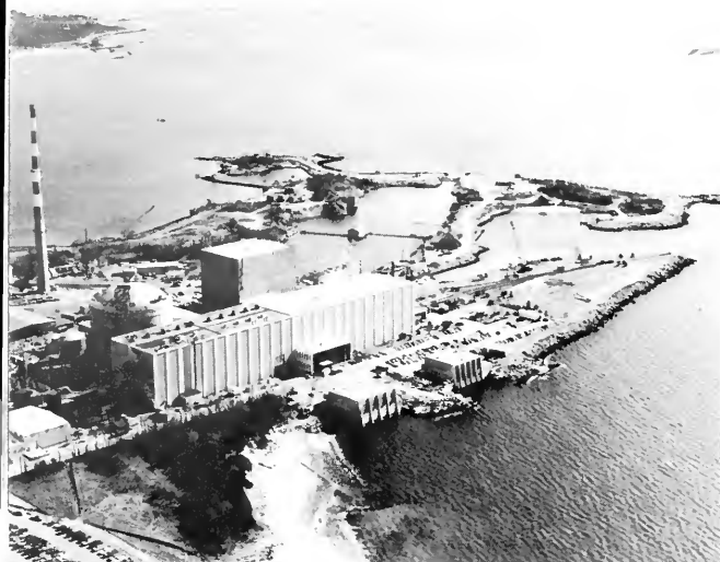
Millstone Point nuclear power station, units 1 and 2. At lower right are two intake structures; at right center is effluent pond; at upper right center is discharge from effluent pond. (Courtesy of Millstone Point nuclear power station, Northeast Utilities)
