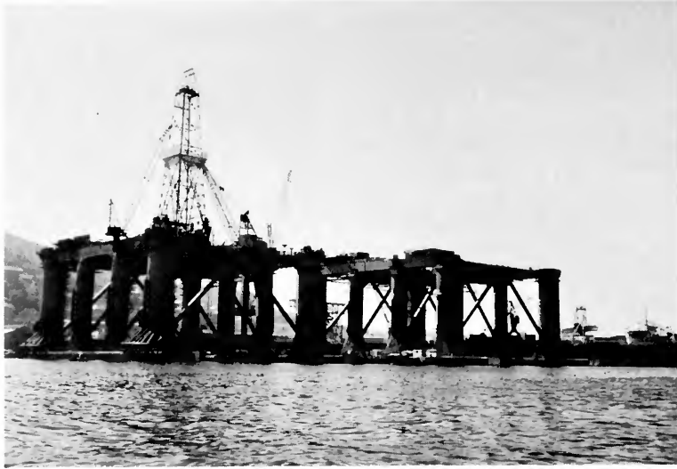
Oil rigs under construction, Bergen, Norway. (Richard Allen)
