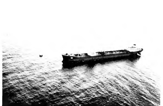
Figure 13. Tanker loading crude oil from production through SALM.
