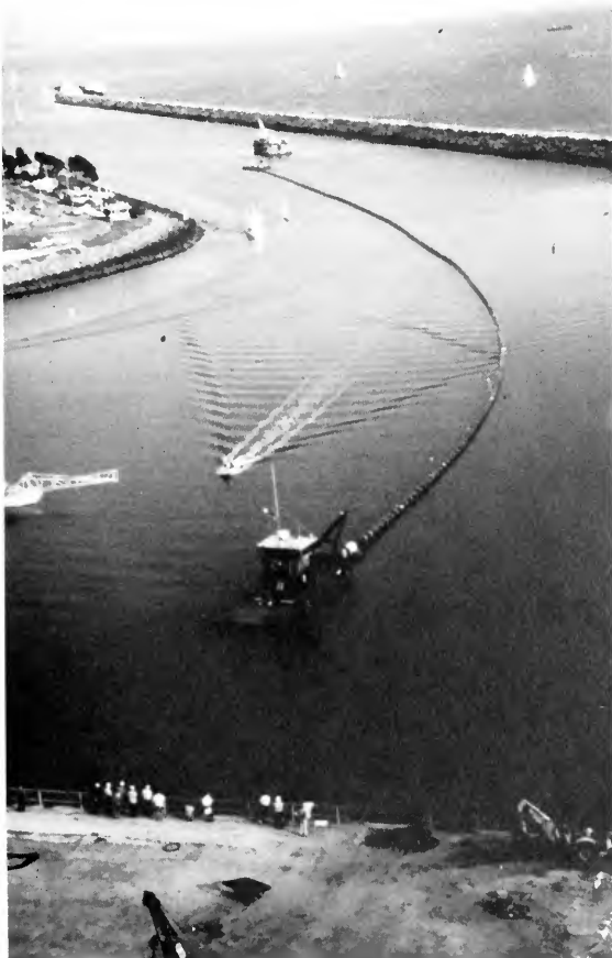
Upwelling pipe being towed to sea.
