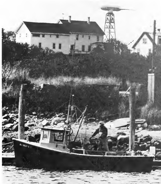
Wind power comes to Block Island, Rhode Island. The single large experimental wind turbine at top of hill was dedicated on June 15, 1979. It is capable of supplying 5 to 15 percent of the island's electricity, or more than $30,000 a year in fuel costs. It is the first federal government wind turbine on the East Coast, a preliminary step toward the production of electric power from locally available resources. It would take from 6 to 20 of these machines to make the island population self-sufficient in electricity. (DOE photo by Dick Peabody)
