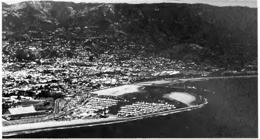
Figure 5. Santa Barbara, California, presents a notable example of longshore sand entrapment by a coastal structure and resultant severe erosion of downdrift beaches.
