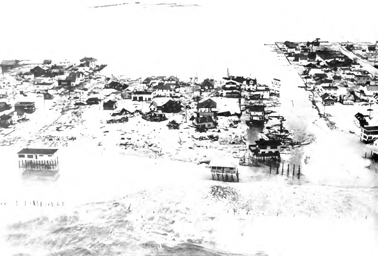
Figure 5. This inlet at Harvey Cedars on Long Beach Island, New Jersey, formed in the 1962 Ash Wednesday storm as a result of a back side development. New inlets on barrier islands usually form as a result of water rushing out of the lagoon. In this case, the outgoing water flowed into a finger canal and thence across the island. (Photo courtesy U.S. Army Corps of Engineers)
