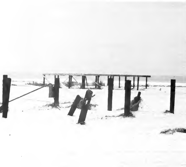
Along a 20-mile reach from Ft. Morgan to Gulf Shores, Alabama, Hurricane Frederic swept hundreds of houses cleanly off their piling foundations. Pilings left behind were often the only evidence remaining that a house had once been on the site. Sand dunes that once fronted the Gulf were flattened and spread hundreds of meters inland.
