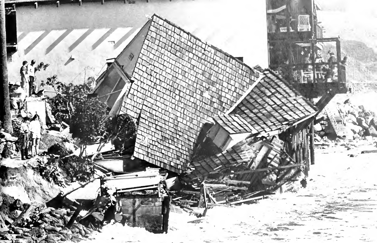
The winter of 1982-83 brought several damaging storms to southern California. Scenes like this will be more common in the future if the expected rise in the atmospheric carbon dioxide content causes sea level to rise. (Los Angeles Times photo)
