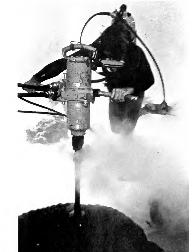
A United States Geological Survey technician operates an underwater drill in order to determine the geological history of an island. (Photo courtesy of University of Miami)
