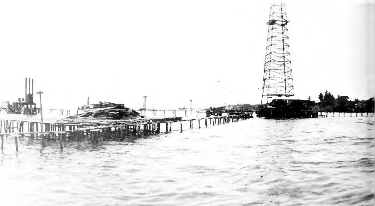
Lagunillas field in Lake Maracaibo, Venezuela, circa 1930. This project was the model for offshore-technology development. (Photo by C. C. McDermond/World Oil)
