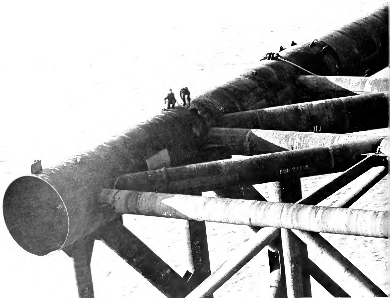
A 4,000-ton drilling platform is readied for sinking to the bottom of the middle ground shoals of Cook Inlet, Alaska. (Photo by Joe Rychetnik/PR)
