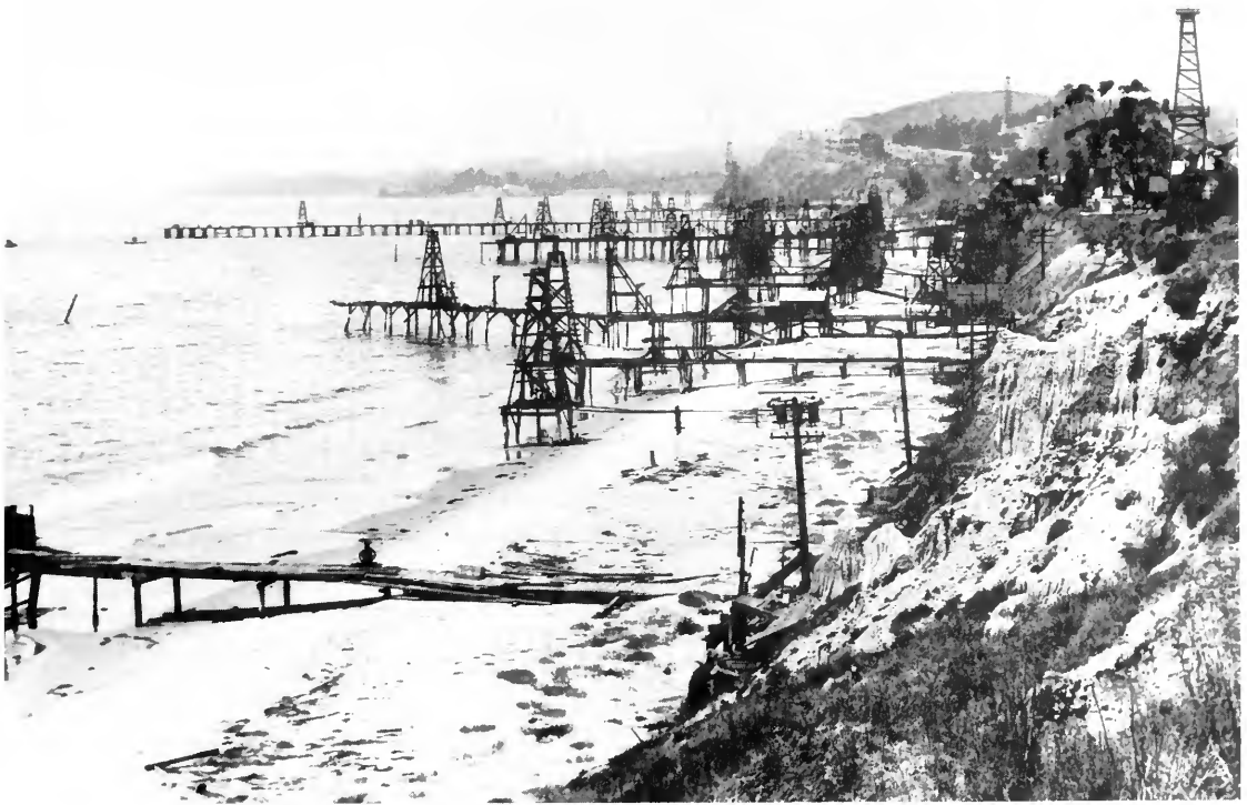
Among the first wells drilled over water were these located on piers in the Summerland field, California, just south of Santa Barbara. This 100-acre field produced from a depth of 210 feet. The photo was taken circa 1920. (Courtesy of World Oil)
