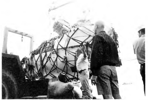
The low point in Alvin's career was from October 1968 to September 1969, when it sank to 5,040 feet near Hydrographer Canyon, south of Nantucket. At left, Alvin on the bottom, as photographed by the U.S. Navy's Mizar. At right, when Alvin was hoisted to within 50 feet of the surface, divers wrapped these harnesses around it for the tow to Martha's Vineyard. (WHOI archives)
