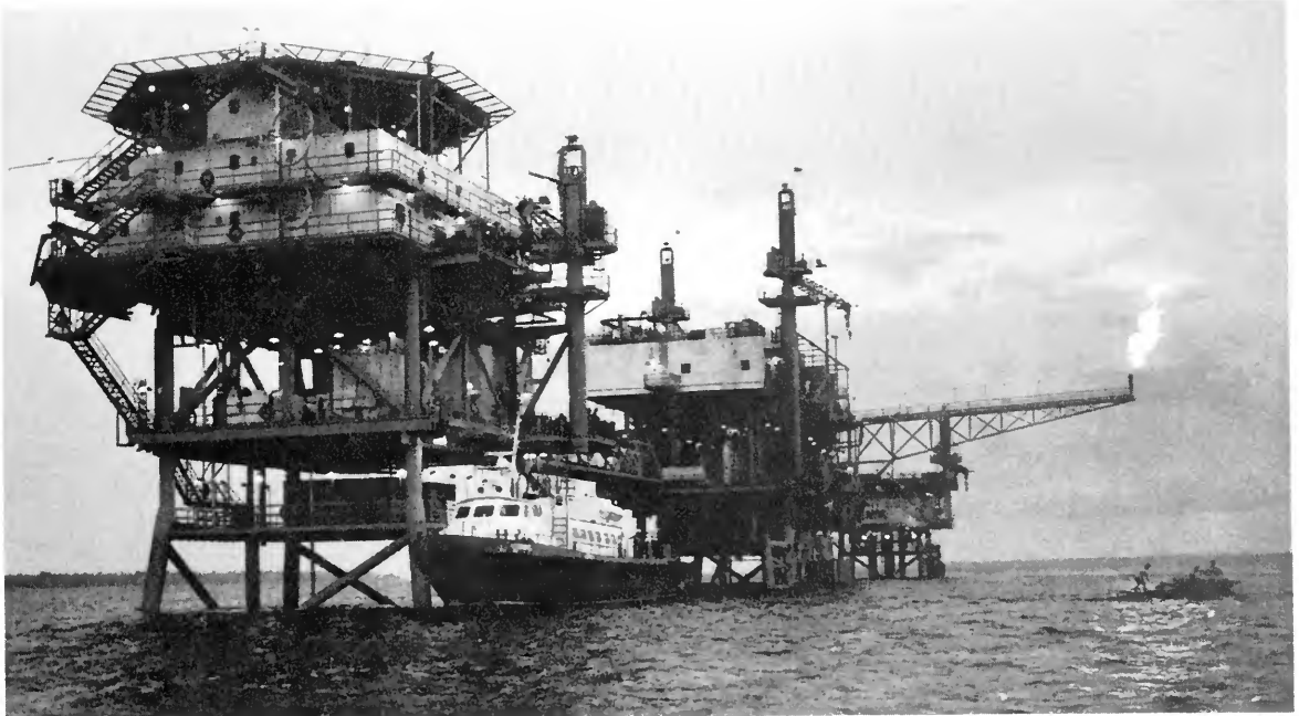
An oil rig with living quarters, production platform, and wellhead platform (at end) in the Lalang oilfield. The Indonesian State Oil Company, Pertamina, contracted this island and surrounding offshore acreage in the Strait of Malacca to Hudebay Oil, Ltd. for commercial oil drilling. (Eurasia Media Co., Ltd.)
