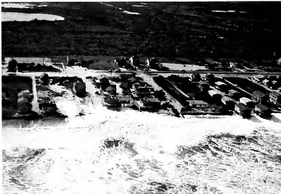
STORM SURGE —The ocean rushes onto the streets of South Nags Head, N.C., wiping out dunes and damaging houses during the “perfect storm” of 1991. Ocean waters wash over barrier islands during storms because winds push water against the shore, low atmospheric pressure allows water levels to bulge upward, and breaking waves force water toward the shore.
