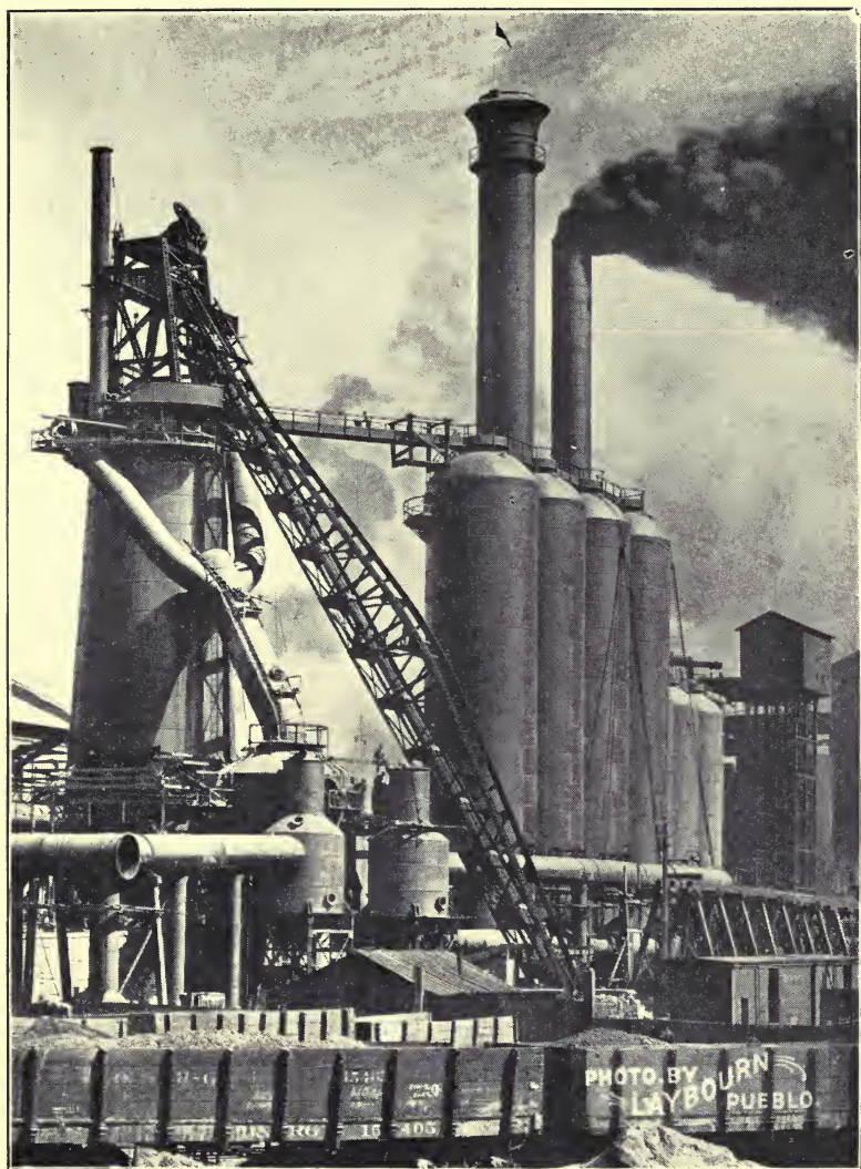
FIG. 100. IRON BLAST-FURNACE.
