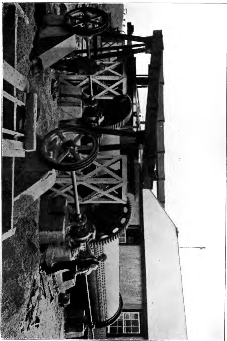
FIG. 68. GATES TUBE MILL.
