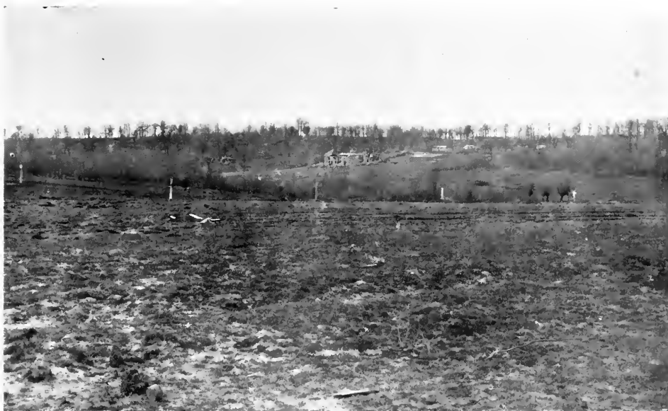
THE MADELEINE FARM AS SEEN FROM THE GROUND WHICH MARKED THE HIGH WATER MARK OF THE 315TH INFANTRY ADVANCE
