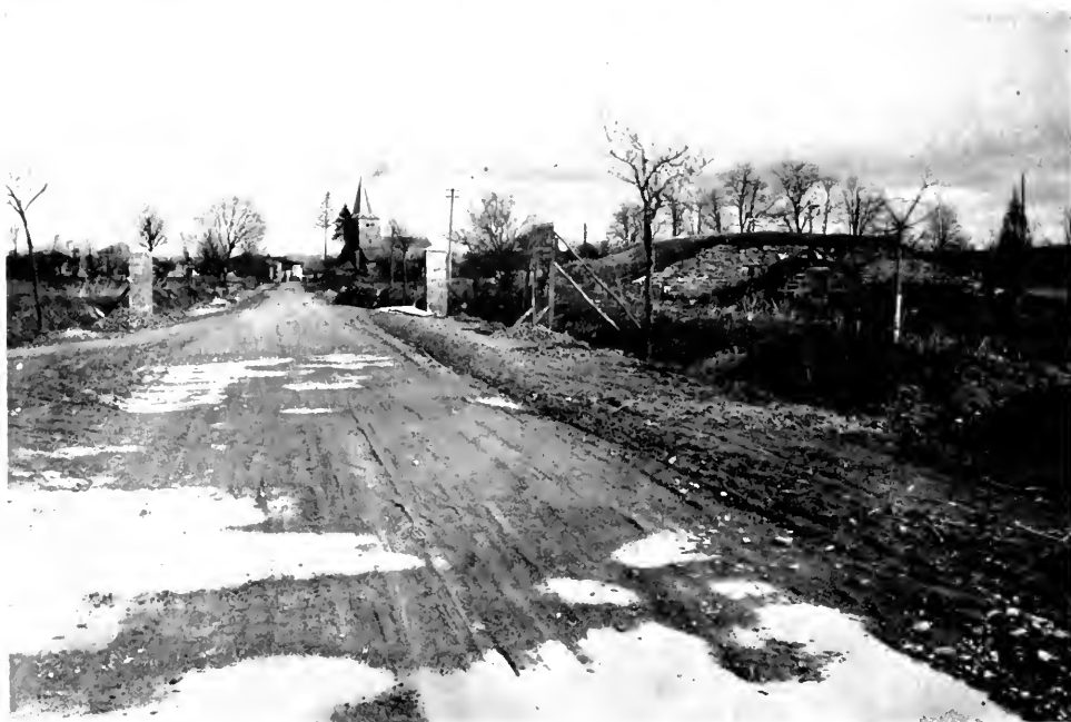
THE ENTRANCE TO DAMVILLERS SHOWING CONCRETE POSTS PUT UP BY THE GERMANS AS TANK OBSTACLES
