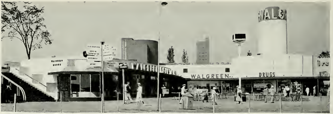
Walgreen Building With Revolving Tower
