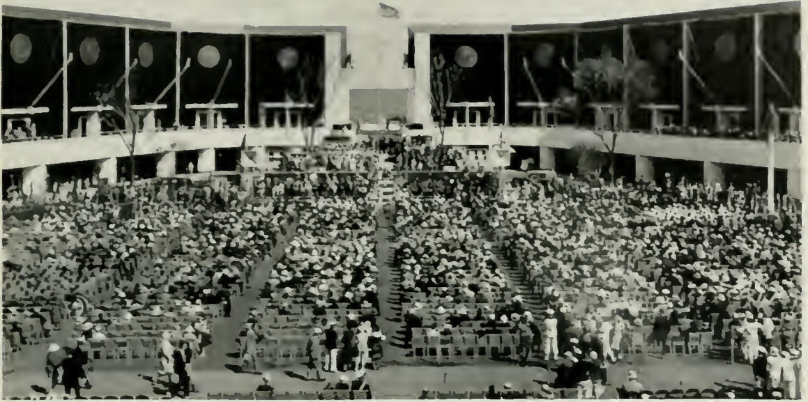
Court of the States Building
