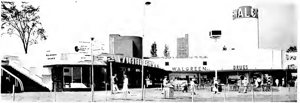
Walgreen Building With Revolving Tower
