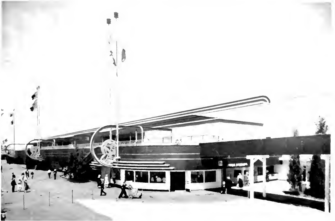
The Food and Agricultural Building—Looking North
