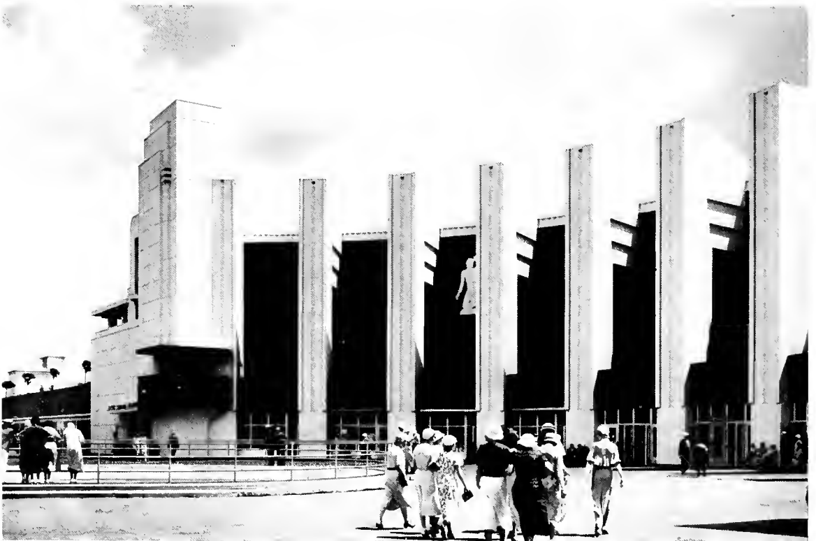
North Facade—The Hall of Science
