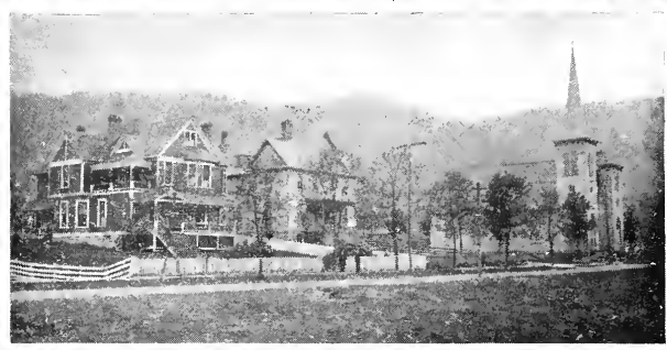
BIG STONE GAP DISTRICT PARSONAGE STATION PARSONAGE AND CHURCH
