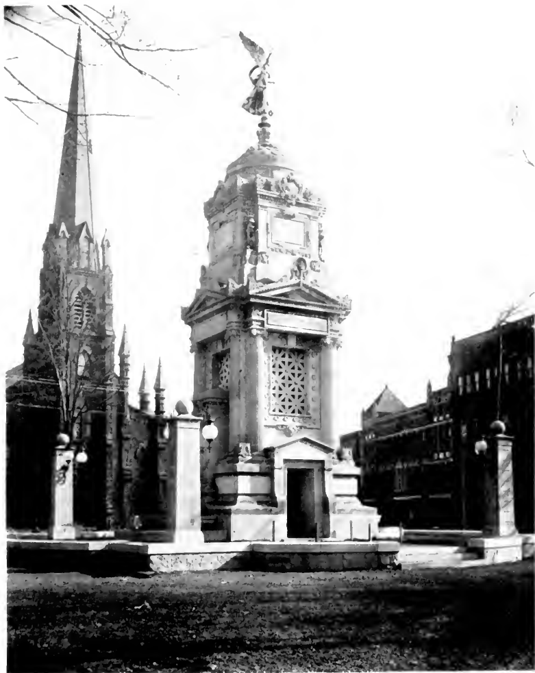
SOUTH VIEW OF MONUMENT.
