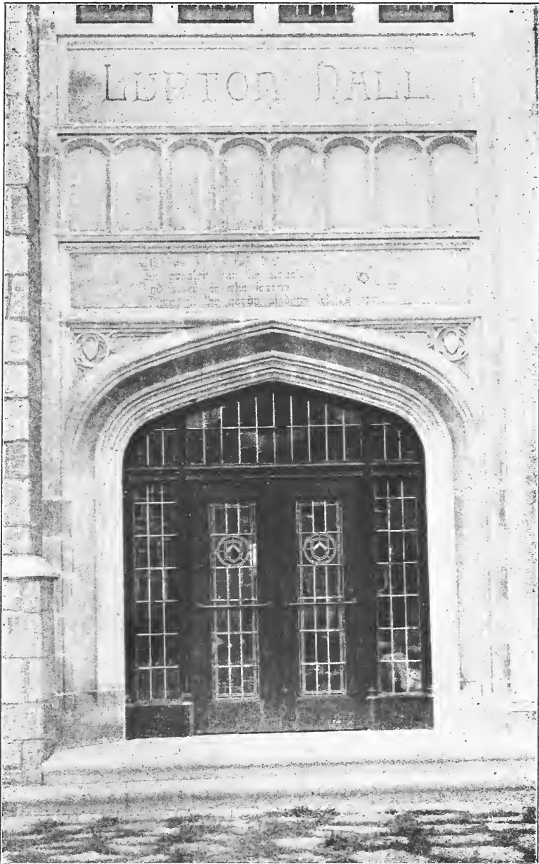
The entrance to Lupton Hall. Above the doorway is engraved the following inscription:
