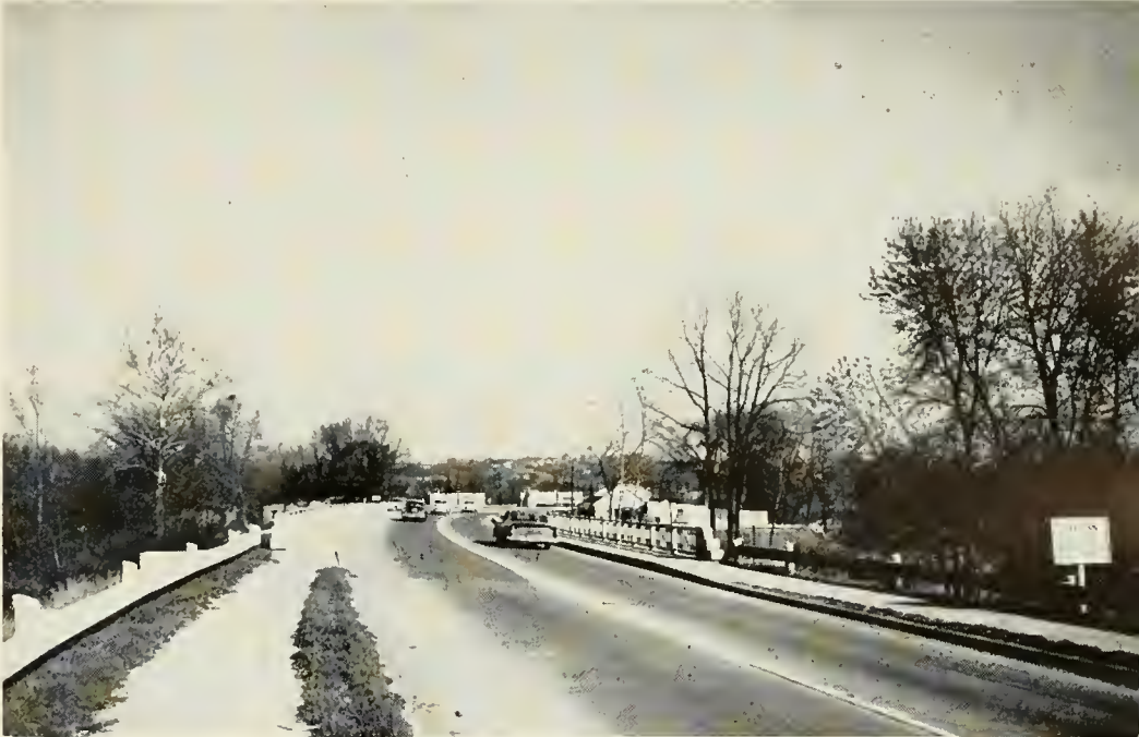
NEW BRIDGE near White's Mill replaced old steel covered structure in major construction project to straighten section of State Route 56.
