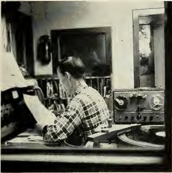
RADIO STATION WATH, located on Route 33 just north of the city, was built in 1950. Announcer is Ted Covert.
