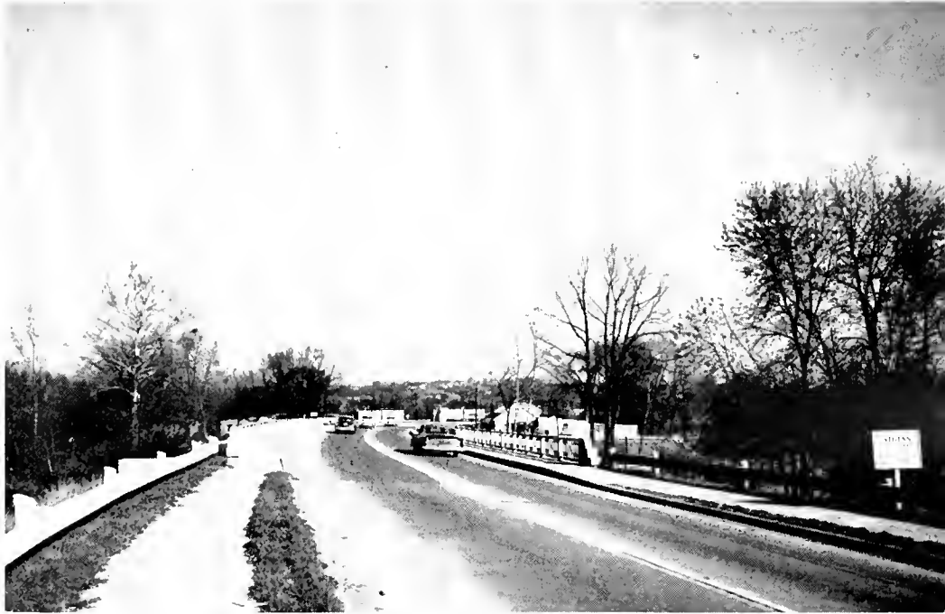
NEW BRIDGE near White's Mill replaced old steel covered structure in major construction project to straighten section of State Route 56.
