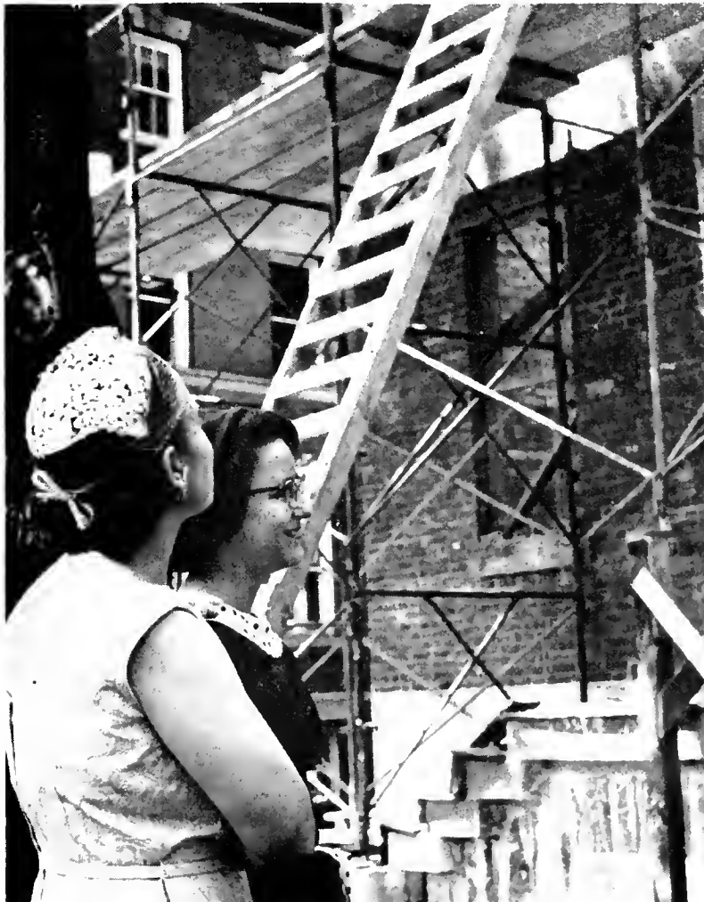
TOUR OF CAMPUS gives mam a chance to see changes which are taking place. Here she and Anita inspect progress at Helen Mauck Galbreath Memorial Chapel.
