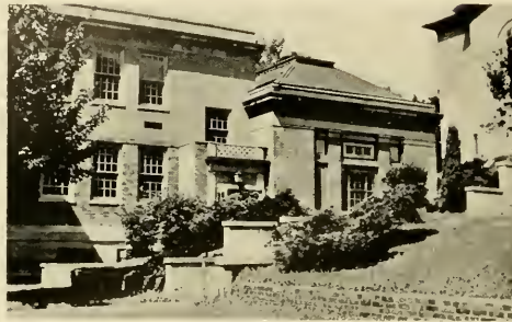
Northeast Entrance, Carnegie Hall
