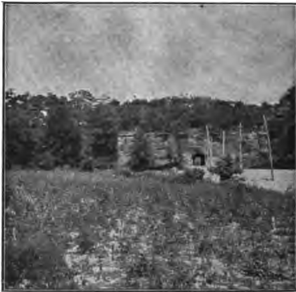
TUNNEL THROUGH RED ROCK, EASTERN BOUNDARY OF OLD CHANNEL.
