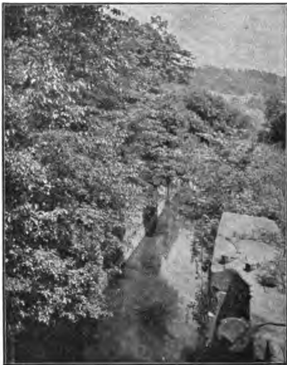
OUTLET LOCK AT HEAD OF "NARROWS."
