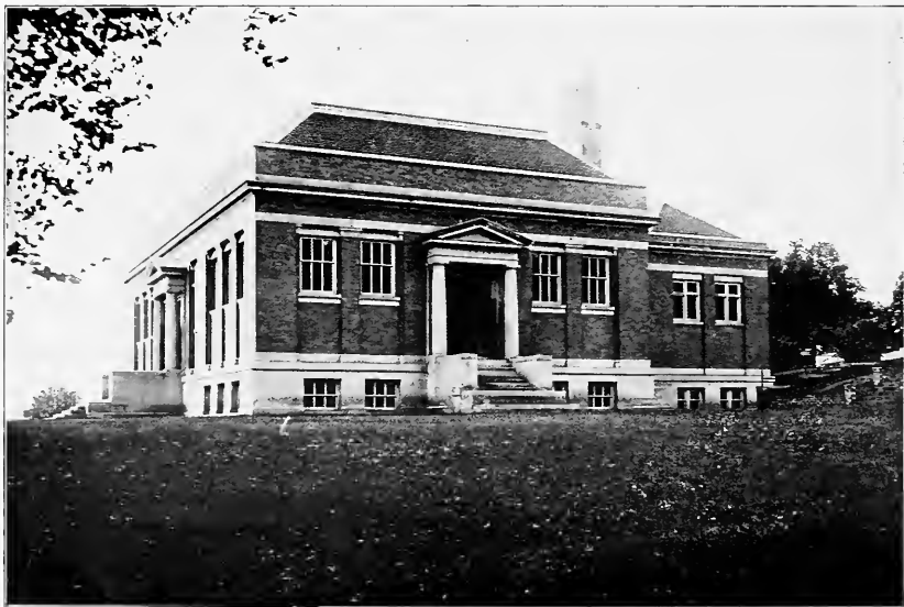
EAST VIEW, CARNEGIE LIBRARY
