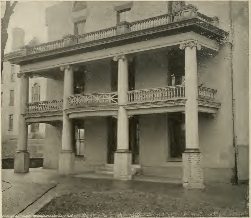
West Wing Portico
