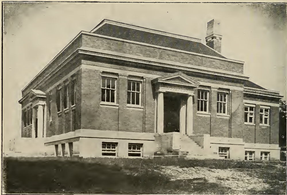
East View, Carnegie Library
