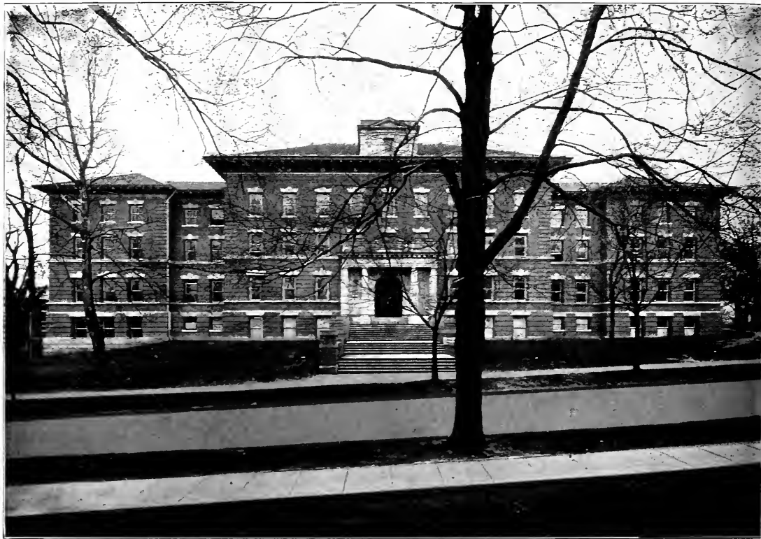
Front View of Ellis Hall
