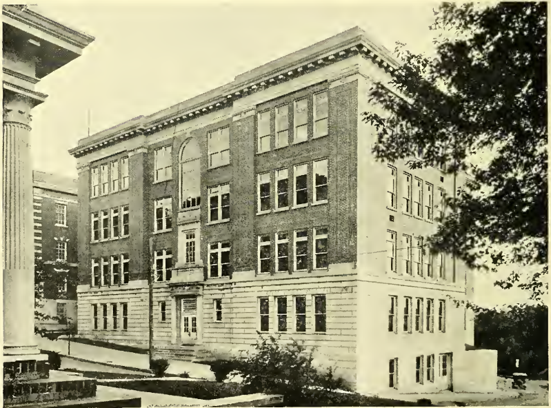
SUPER HALL (ENGINEERING—PHYSICS—INDUSTRIAL ARTS)
