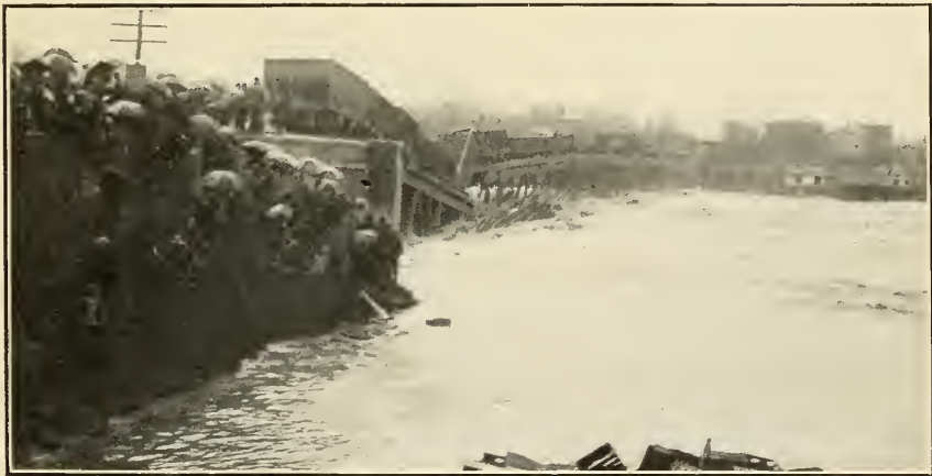
B. DURING FAILURE.
