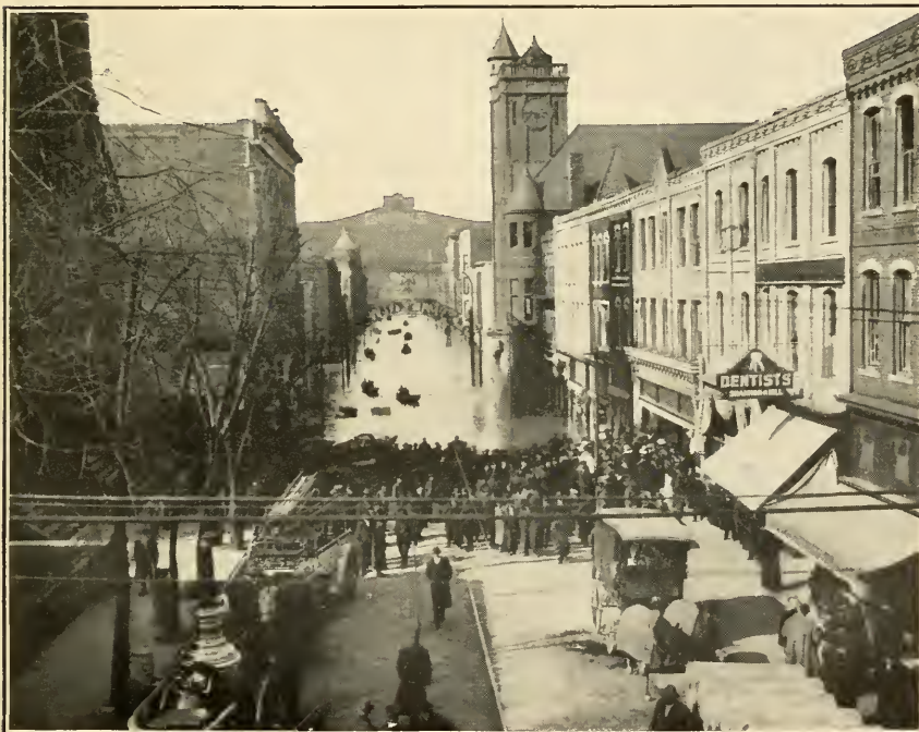
B. MARKET STREET, PARKERSBURG, W. VA., DURING FLOOD OF MARCH-APRIL, 1913.
