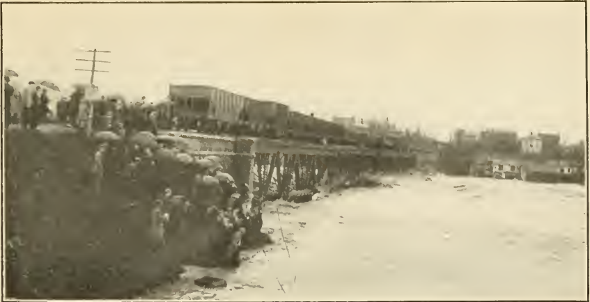
A. JUST BEFORE FAILURE.
