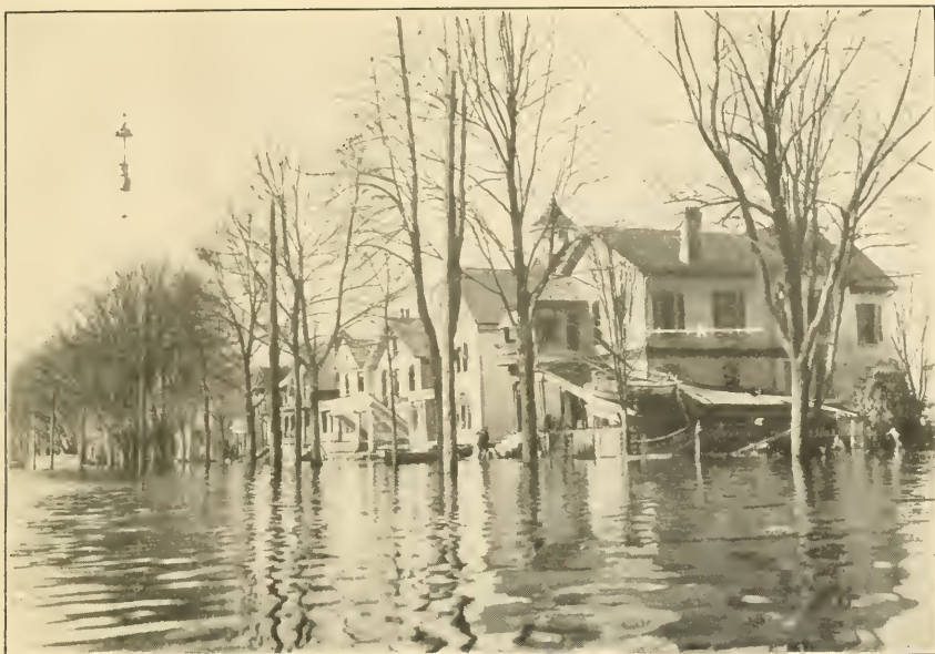
A. SECOND STREET, MARIETTA, OHIO, DURING FLOOD OF MARCH-APRIL, 1913, AFTER WATER HAD FALLEN.
