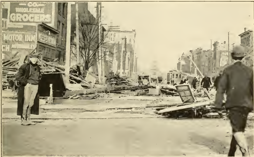
B. SAME STREET AFTER THE FLOOD.
