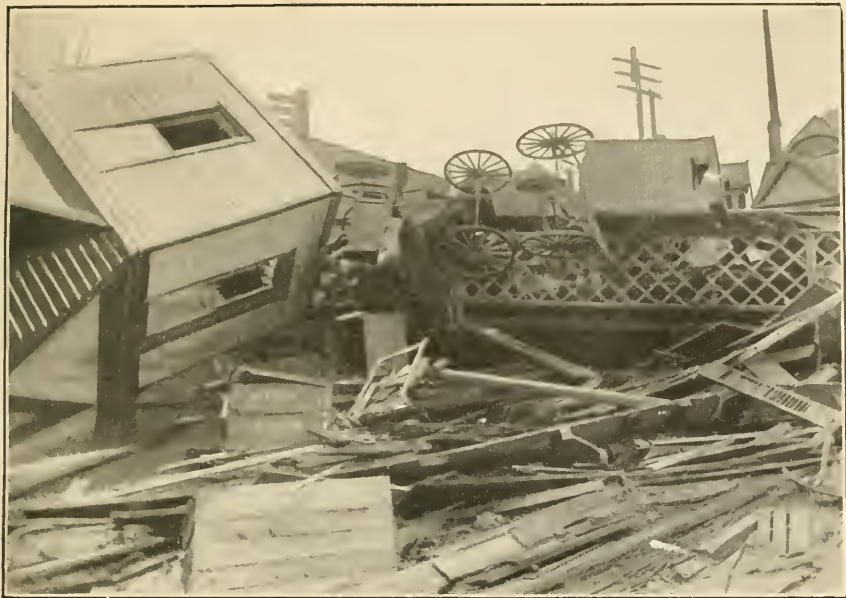
.A. MIAMI STREET CANAL BRIDGE, DAYTON, OHIO, AFTER THE FLOOD OF MARCH-APRIL, 1913.
