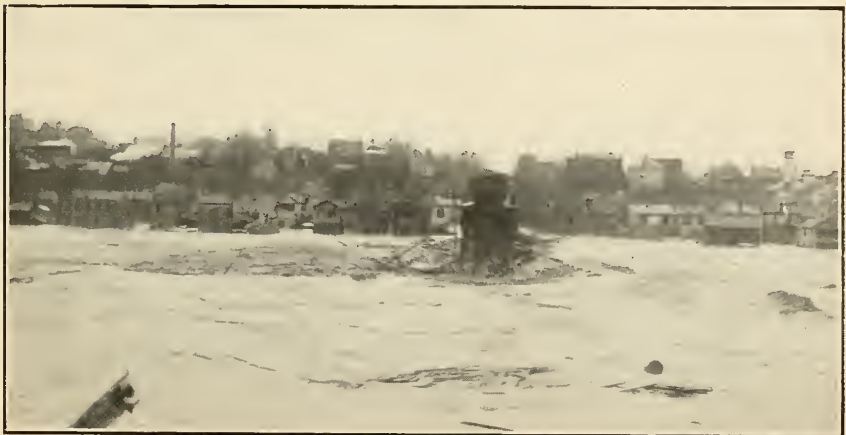
C. IMMEDIATELY AFTER FAILURE.
