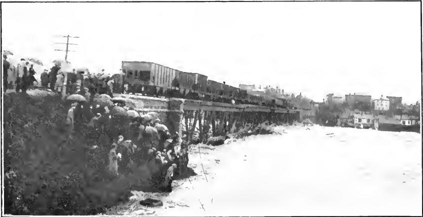
A. JUST BEFORE FAILURE.
