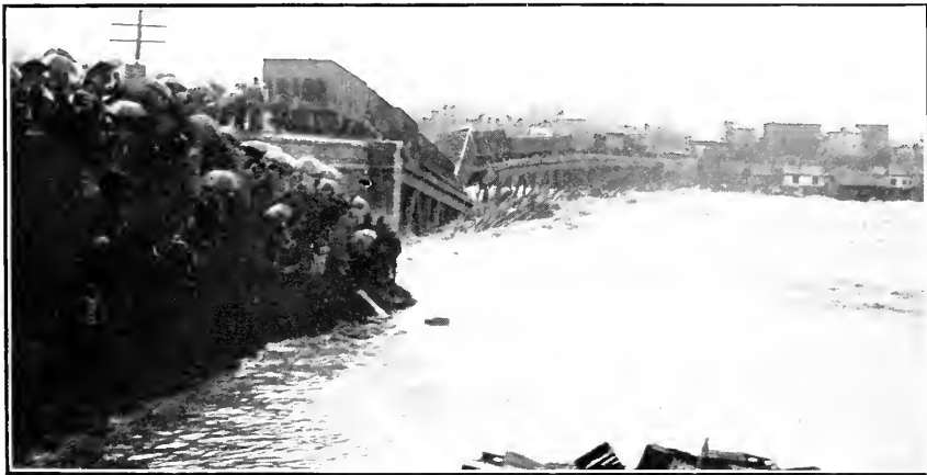
B. DURING FAILURE.
