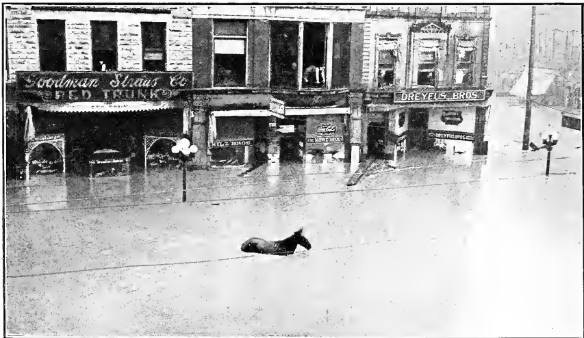
.2. HIGH STREET, HAMILTON, OHIO, DURING FLOOD OF MARCH-APRIL, 1913.
