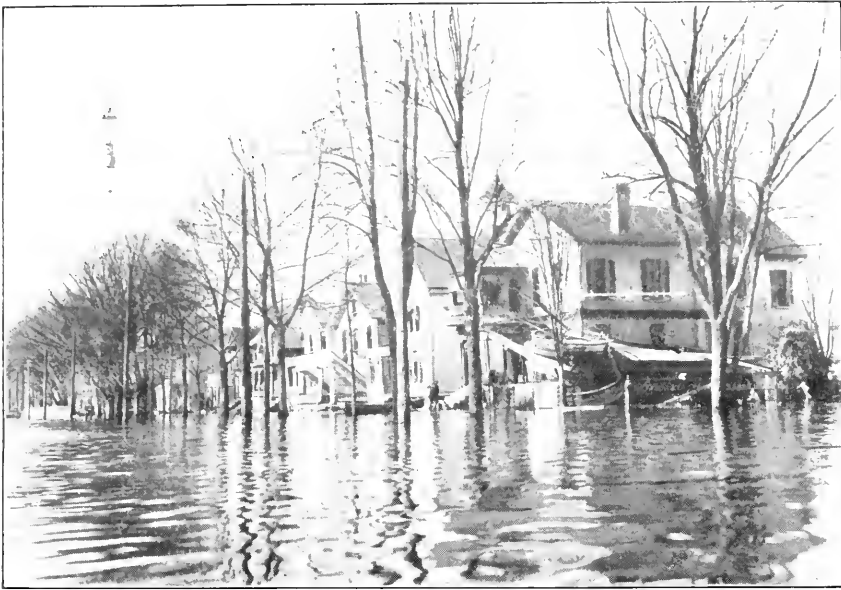
A. SECOND STREET, MARIETTA, OHIO, DURING FLOOD OF MARCH-APRIL, 1913, AFTER WATER HAD FALLEN.
