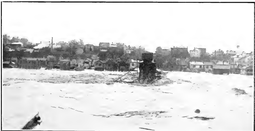
C. IMMEDIATELY AFTER FAILURE.
