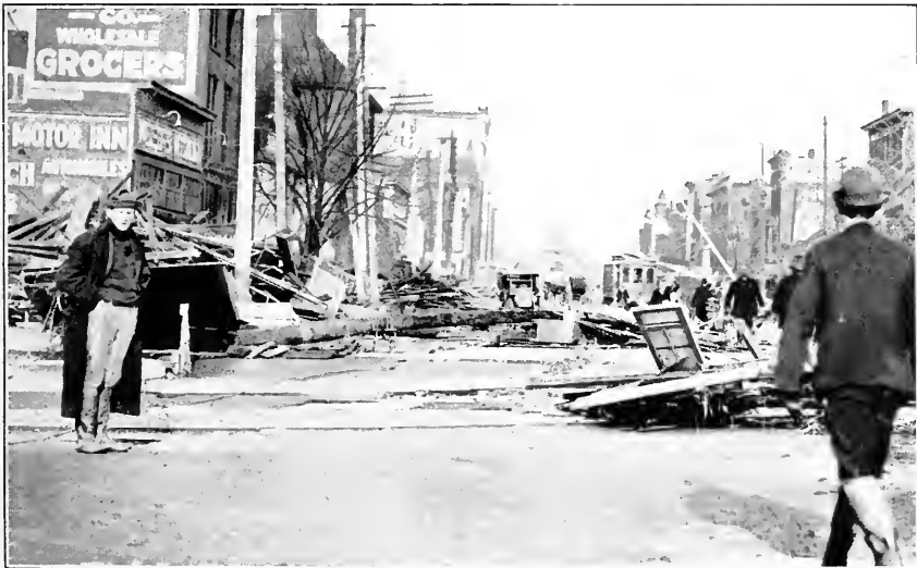
2. SAME STREET AFTER THE FLOOD.
