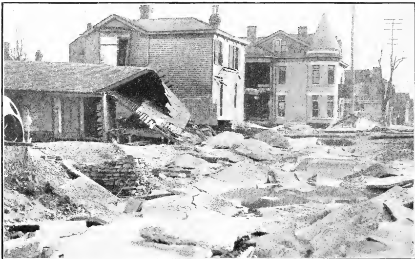
A. SOUTH B STREET, HAMILTON, OHIO, AFTER THE FLOOD OF MARCH-APRIL, 1913.
