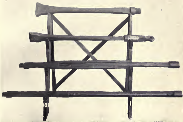
TOOLS USED BY COLONEL E. L. DRAKE IN SINKING THE FIRST PETROLEUM WELL.
