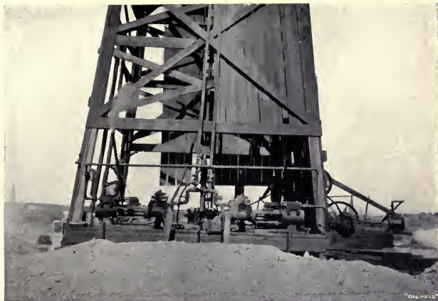
GENERAL VIEW OF A ROTARY DRILLING PLANT.
