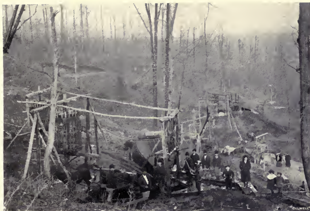
HAND-DUG WELLS IN ROUMANIA.
