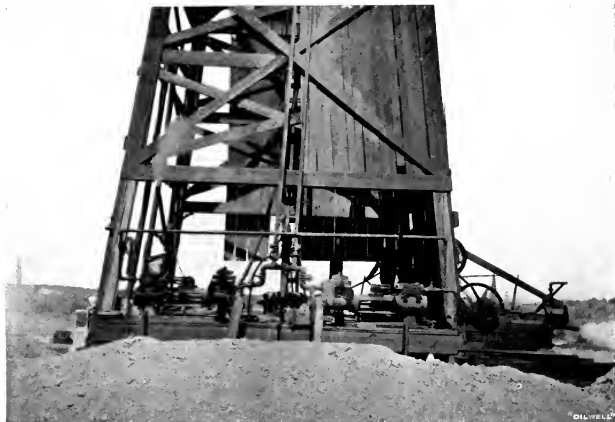
GENERAL VIEW OF A ROTARY DRILLING PLANT.
