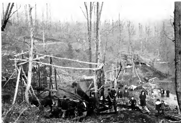
HAND-DUG WELLS IN ROUMANIA.
