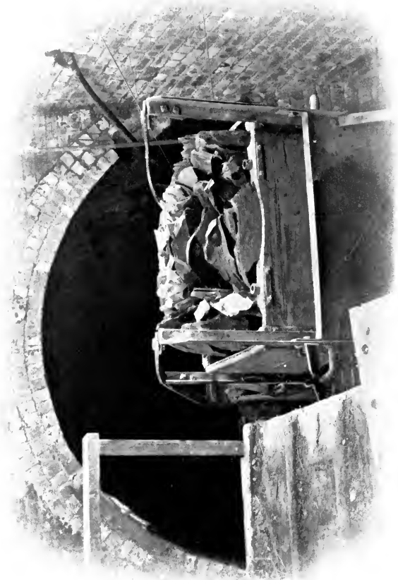
ONE OF THE "HUTCHES" EMPLOYED FOR TRANSPORTING THE SHALE.
