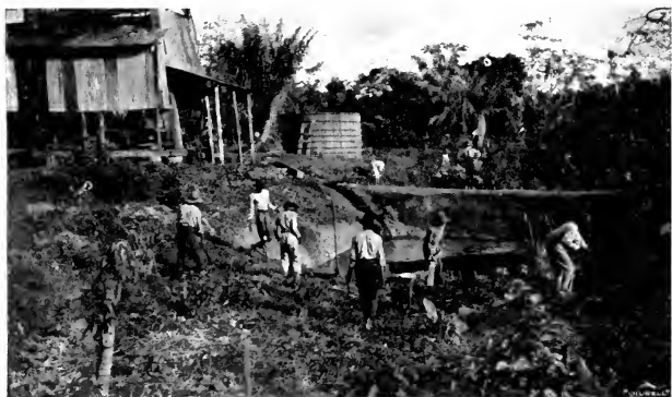
DIGGING A "SUMP" ON A TRINIDAD OIL-FIELD.
