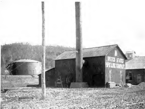
PUMPING-STATION ON THE UNITED STATES PIPE-LINE.
