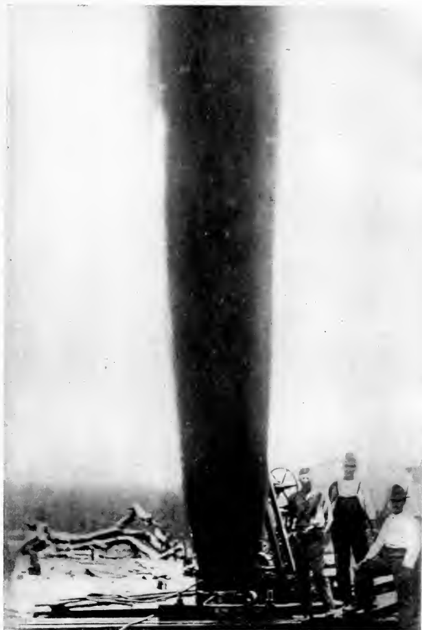
THE FAMOUS POTRERO DE LLANO NO. 4 BLOWING THROUGH THE GATE VALVE.
