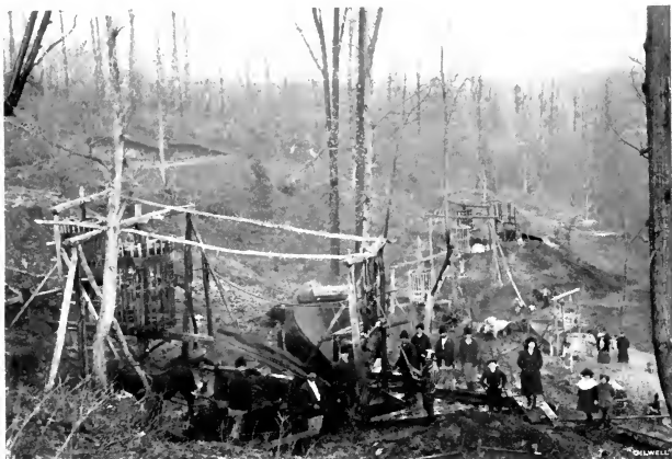
HAND-DUG WELLS IN ROUMANIA.
