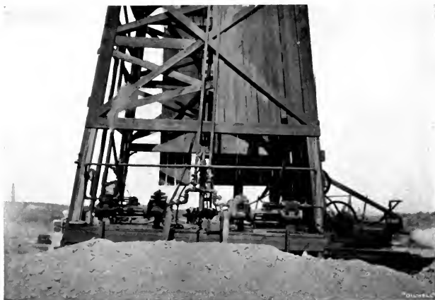
GENERAL VIEW OF A ROTARY DRILLING PLANT.
