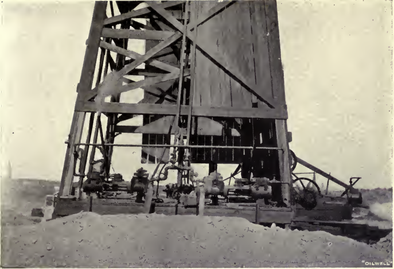
GENERAL VIEW OF A ROTARY DRILLING PLANT.
