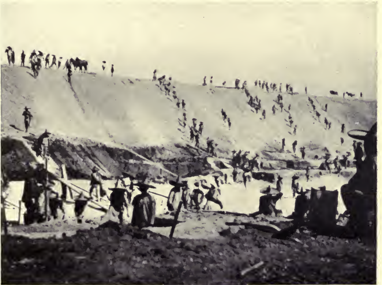
BUILDING THE EARTH RESERVOIR TO RECEIVE THE FLOW FROM POTRERO DE LLANO NO. 4.
