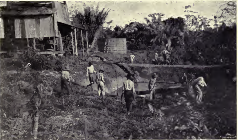
DIGGING A "SUMP" ON A TRINIDAD OIL-FIELD.
