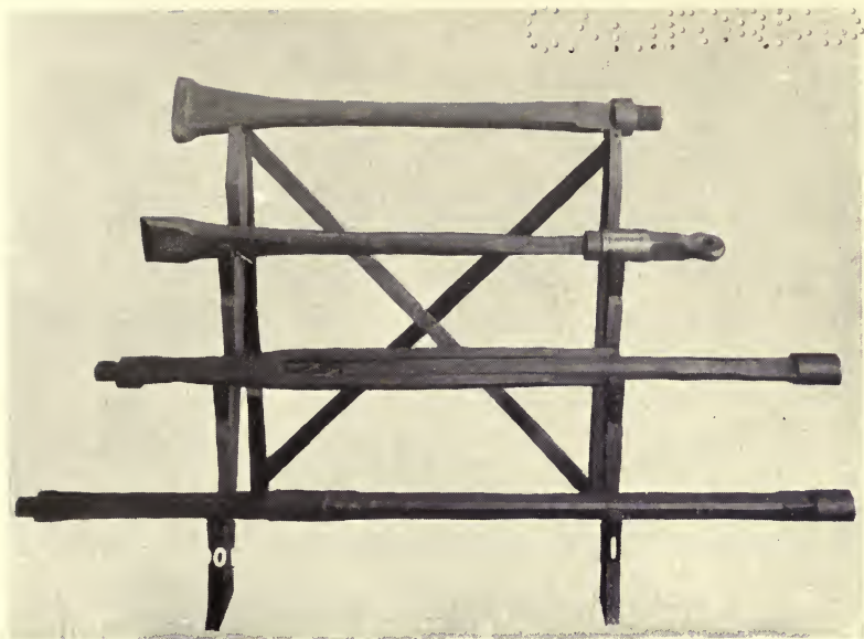
TOOLS USED BY COLONEL E. L. DRAKE IN SINKING THE FIRST PETROLEUM WELL.
