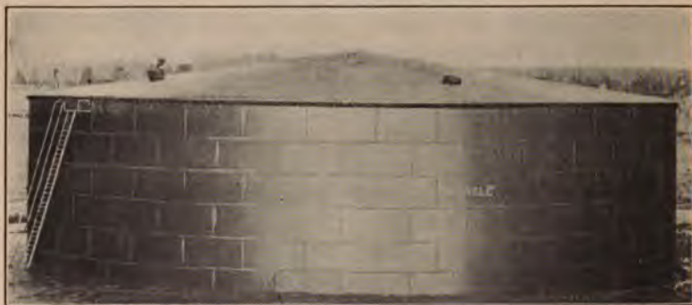
FIG. 68.—Steel storage tank of 37,500 to 50,000 bbl. type.
