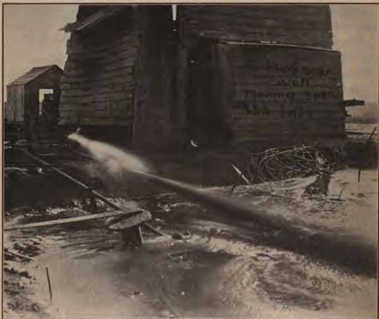
FIG. 40.—Burkwaggoner well at Burkburnett, Texas, flowing 3000 bbls. per day through flow line. (Courtesy Los Angeles Chamber Mines and Oil.)
