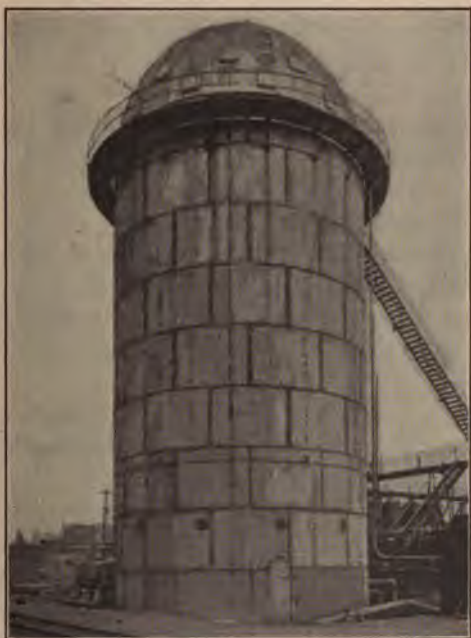
FIG. 92.—Five thousand bbl. illuminating oil agitator in which the crude kerosene is chemically treated and washed with water, air being used to agitate the oil during treatment. (After C. W. Stratford.)
