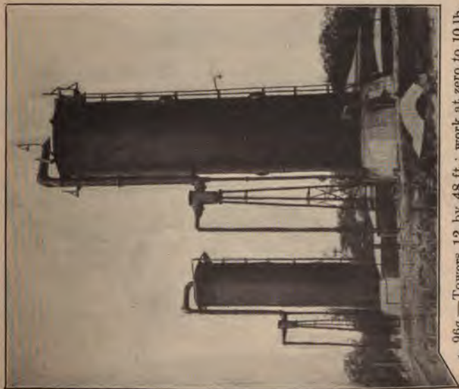
FIG. 96b.—Gas intake side of high pressure absorption towers. (After U. S. B. M.)
