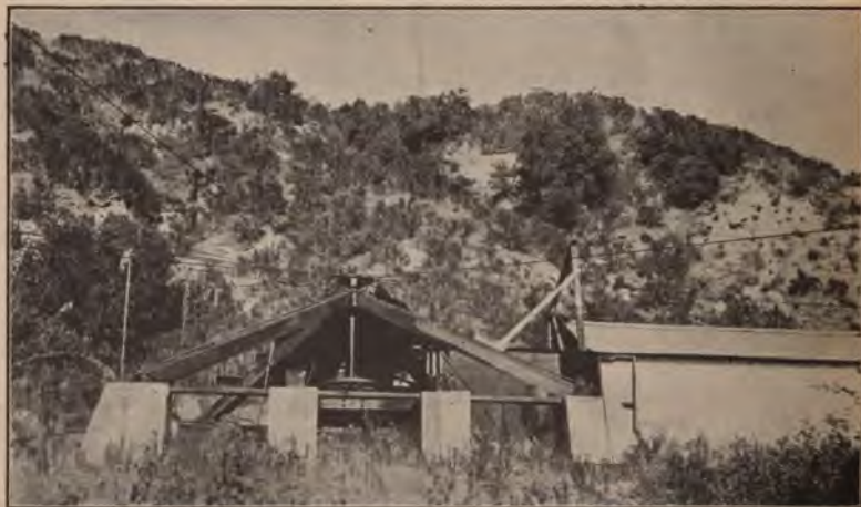
FIG. 48.—Pumping power using wire cables, Newhall, Calif.
