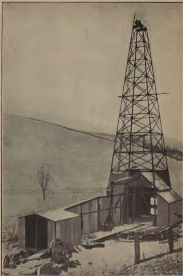
FIG. 5.—Steel derrick for drilling or for pumping wells.
