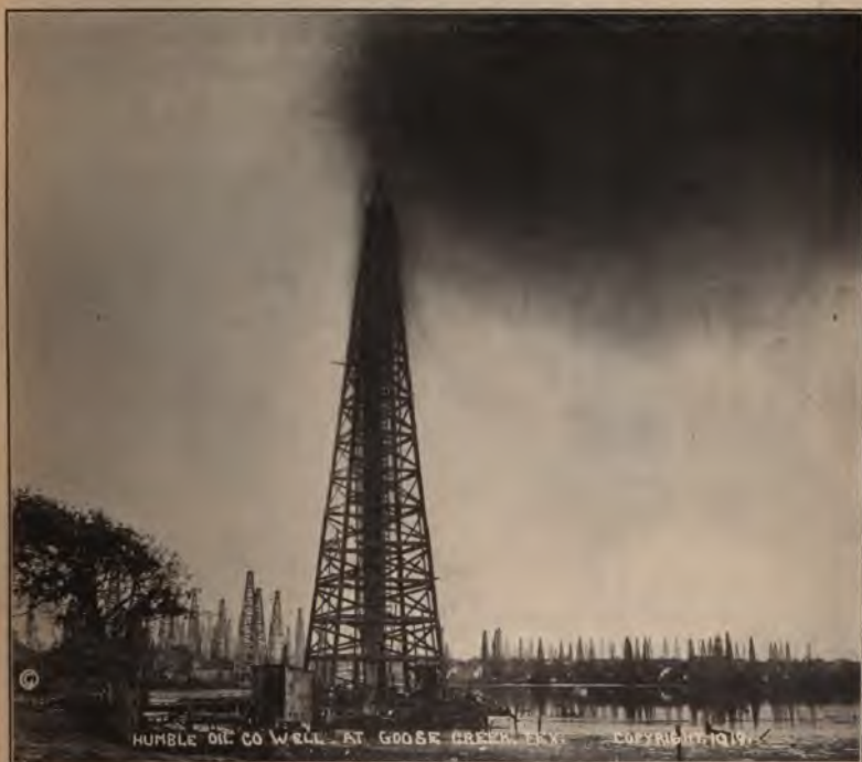
FIG. 41.—Flowing well of Humble Oil Co. at Goose Creek. (Courtesy Los Angeles Chamber Mines and Oil.)
