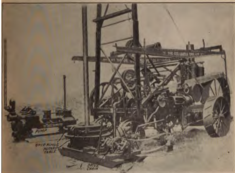
FIG. 4.—Portable rotary-drilling rig.
