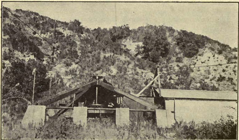
FIG. 48.—Pumping power using wire cables, Newhall, Calif.
