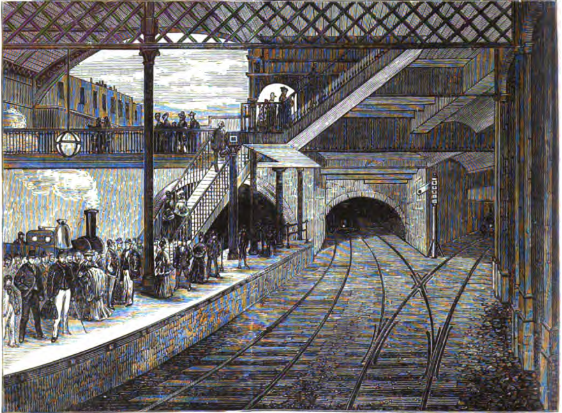
KING'S CROSS UNDERGROUND STATION IN 1868. (See page 227.)
