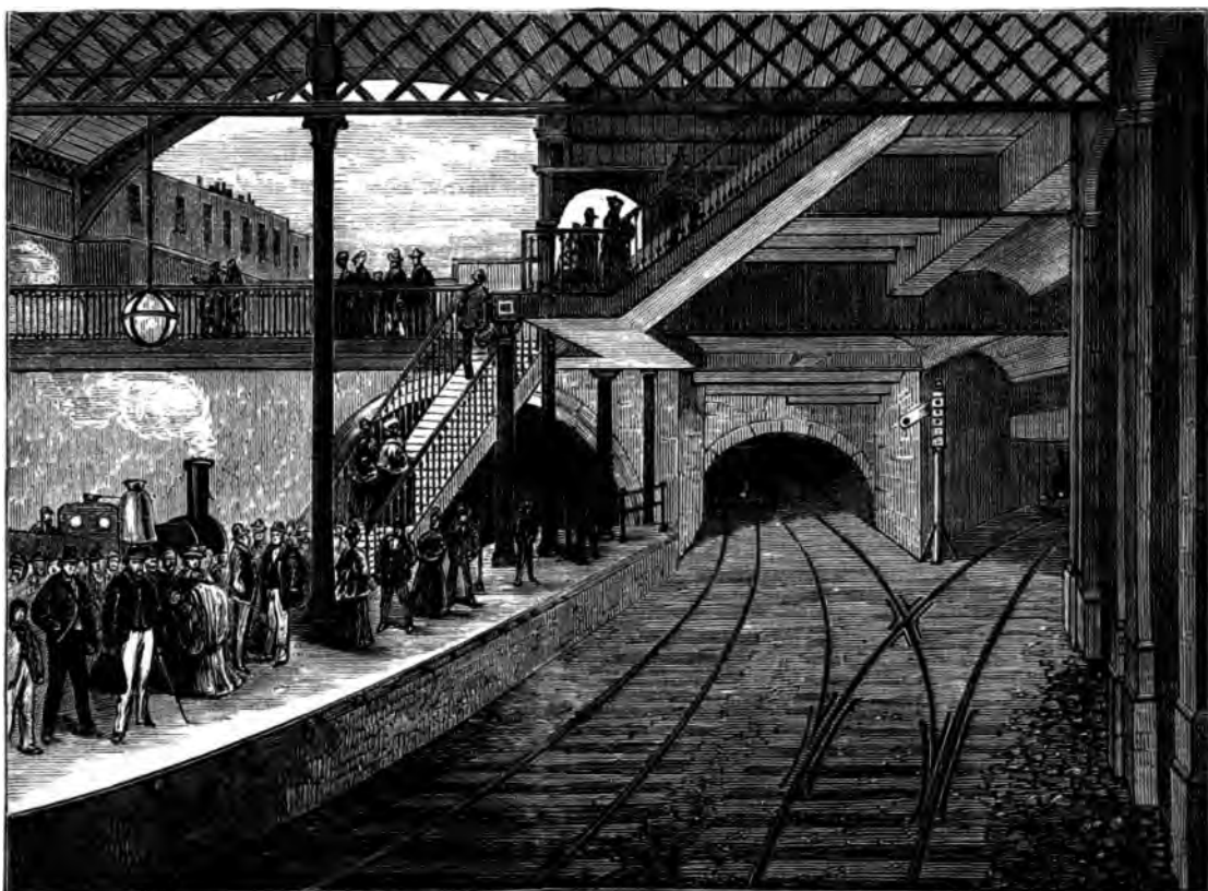
KING'S CROSS UNDERGROUND STATION IN 1868. (See page 227.)
