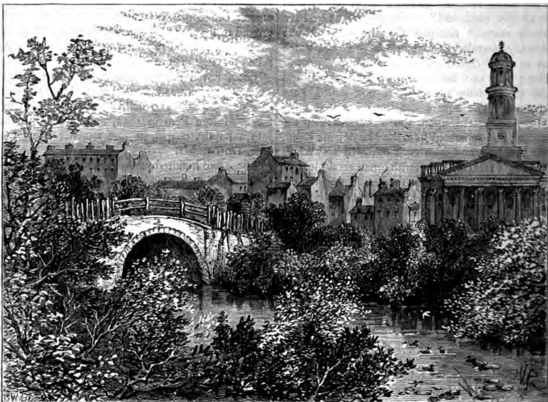
OLD BRIDGE OVER THE LAKE, REGENT'S PARK, IN 1817.
