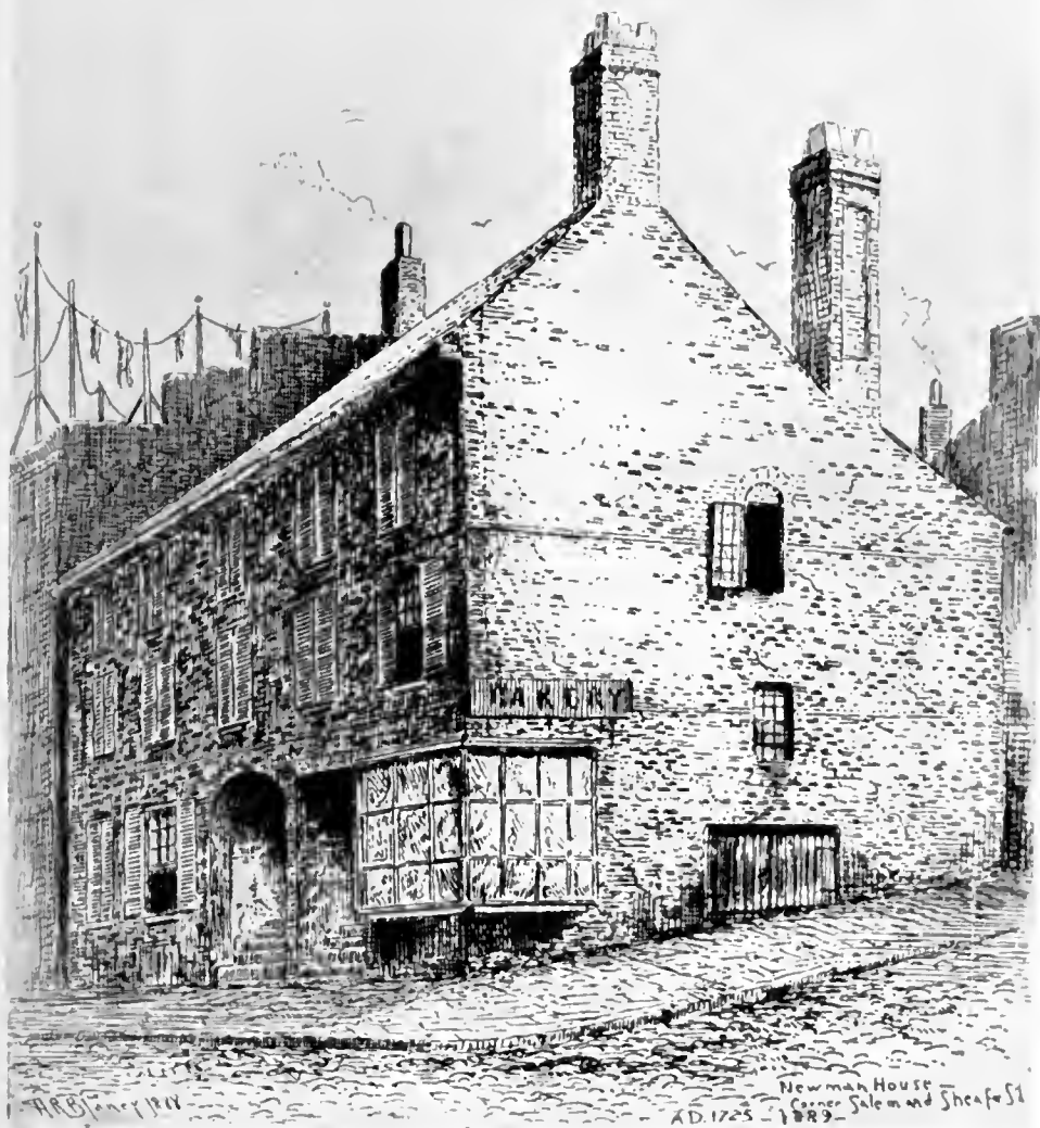
NEWMAN HOUSE, SHEAFE AND SALEM STREETS
