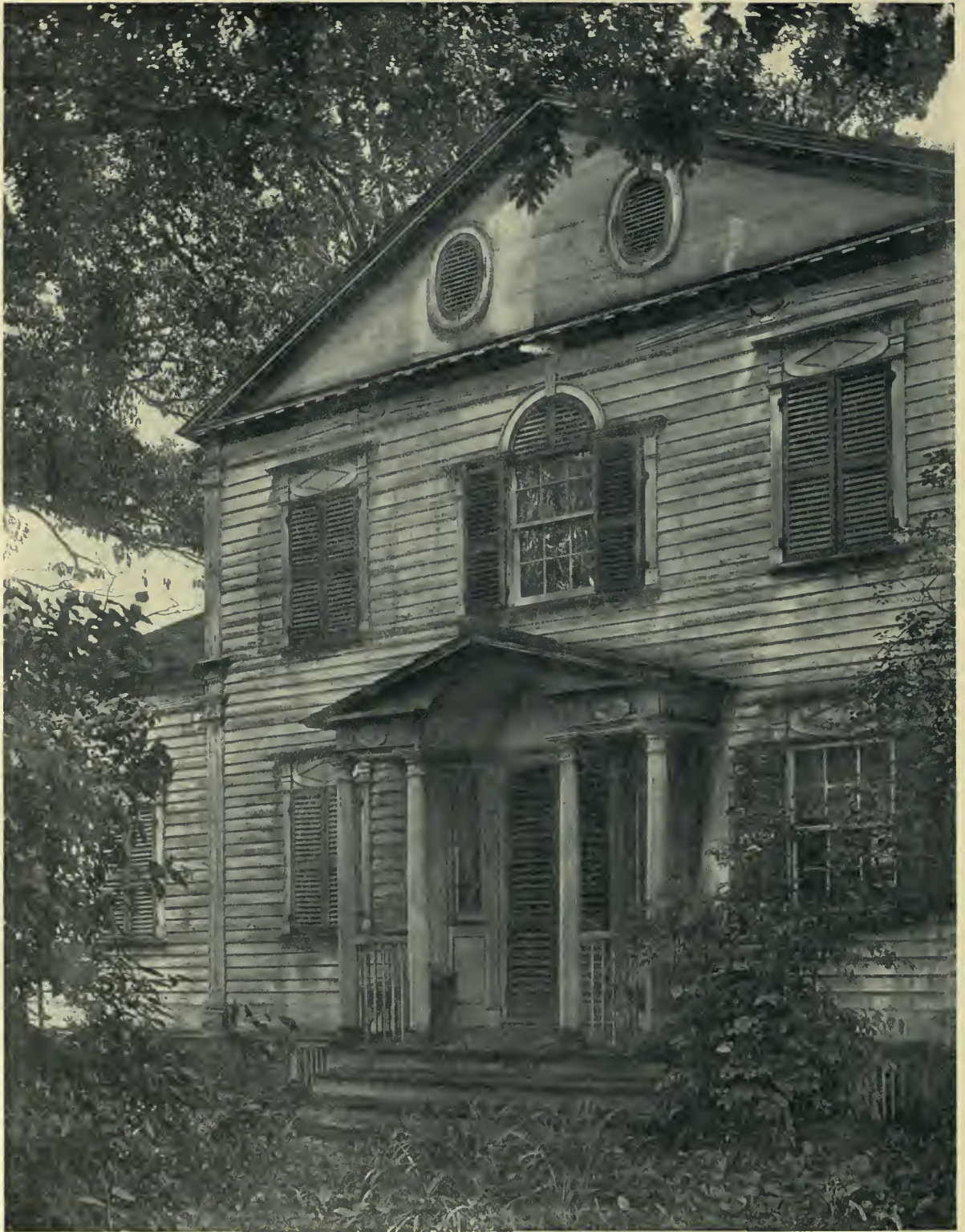
HOUSE AT CHATHAM CENTER, NEW YORK. Detail of Entrance and Front Façade.
