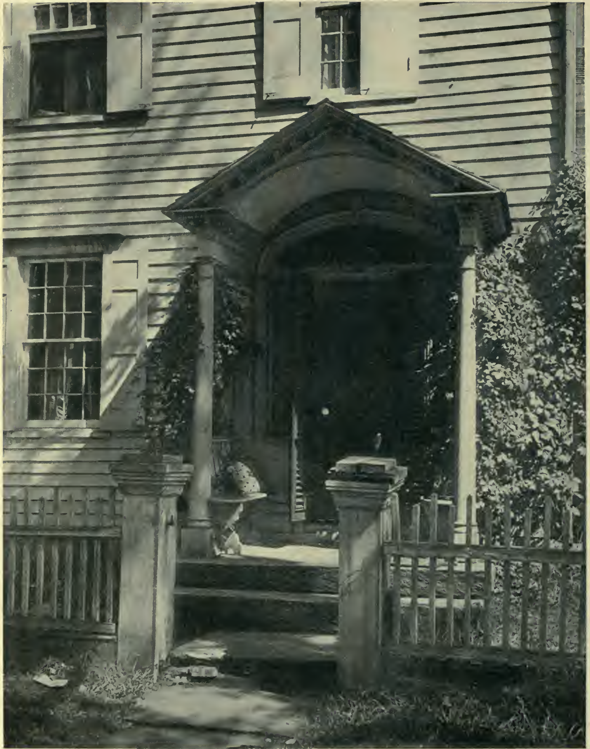
HOUSE IN WEST STREET, DANBURY, CONNECTICUT. Entrance Detail.
